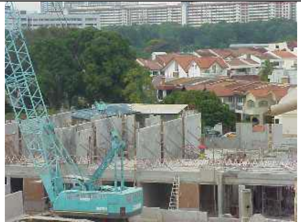
Figure 12.2 Use of 50-tonne crane for hoisting
