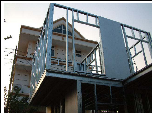
Figure 12.8 Light-gauge Steel Frame
