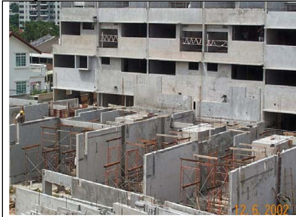
Figure 12.1 Erection of precast walls and planks
