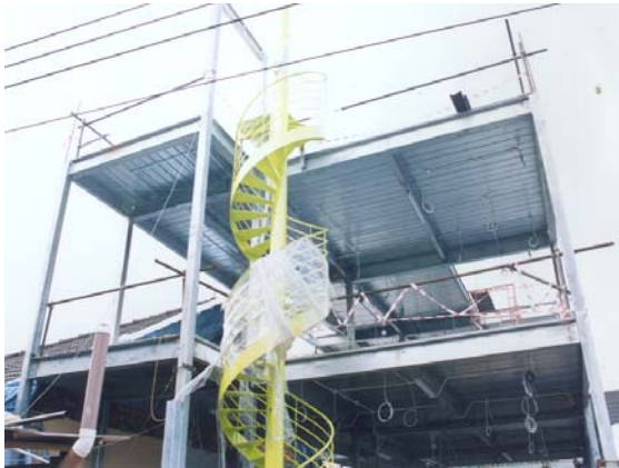
Figure 12.5 Steel decking and prefabricated spiral staircase
