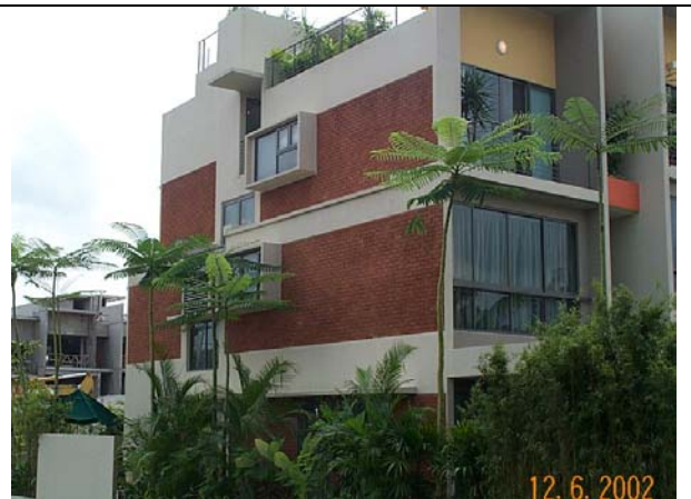
Figure 12.4 Elevation of completed houses
