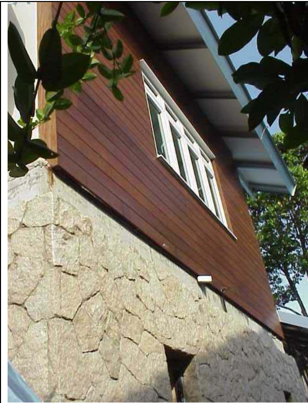
Figure 12.9 External cladding to fibre board walls
