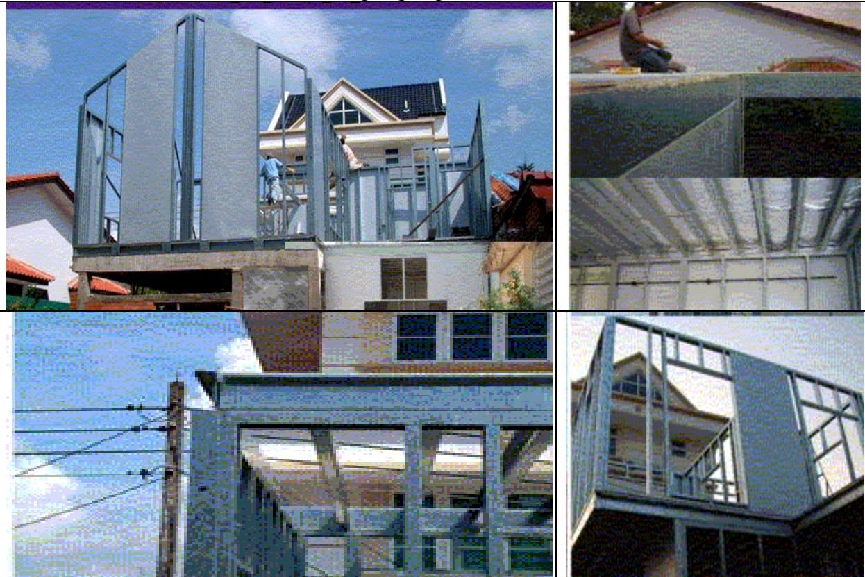
Figure 12.12 Construction of 2 nd storey
