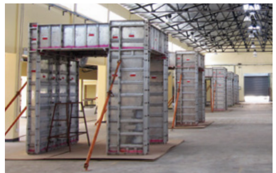
Top | Trainees attending practical training on system formwork at Fonda OTC.
