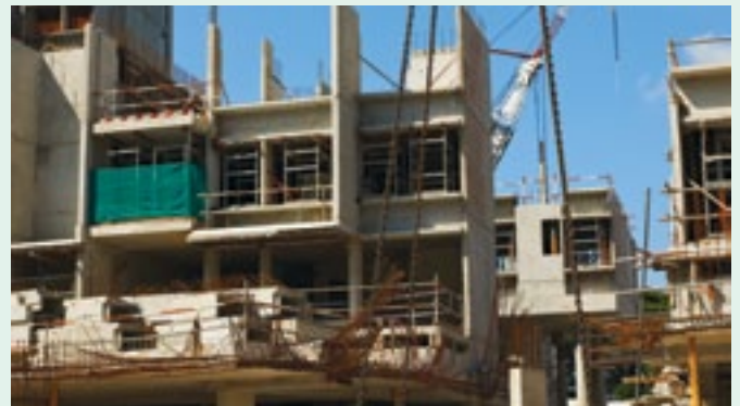
Top | Precast materials allow for faster construction and increase in productivity.
