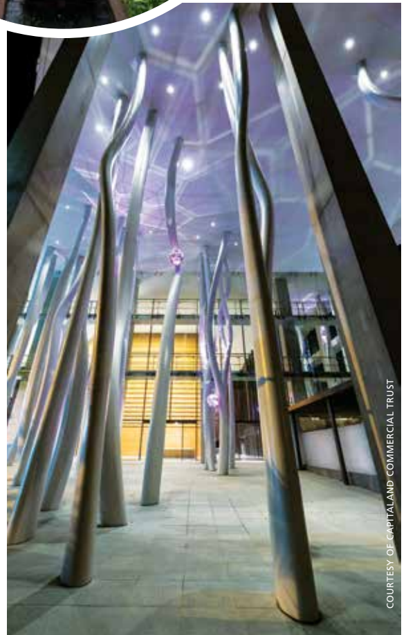
Below: CapitaGreen was the first building to be constructed using ultra-high strength concrete that requires less concrete to be used.
