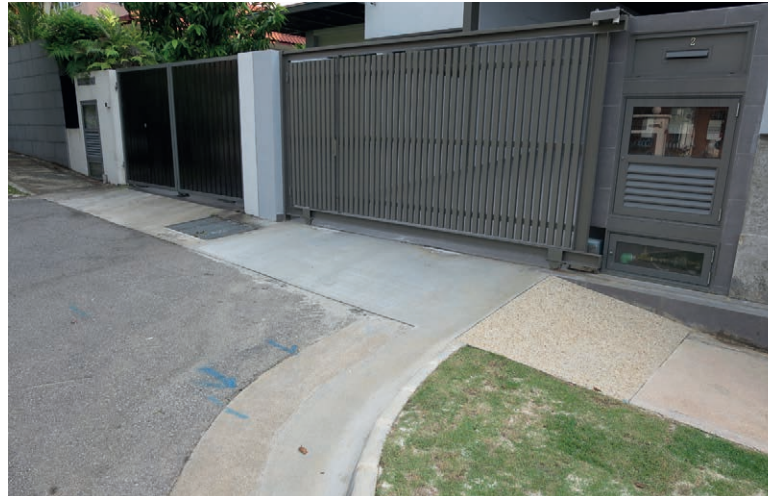
Left: The project needed to meet both PUB's requirement for minimum platform level of the entrance culvert, and LTA's required gradient for the external vehicle ramp.
