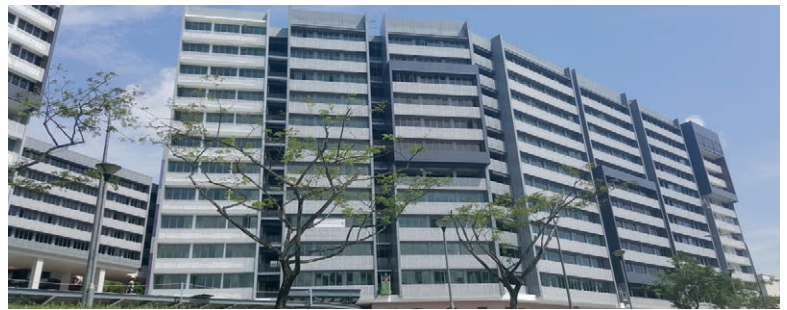
The use of PPVC technology for the new student residences at Nanyang Crescent reduced the construction time and manpower requirements on-site.
