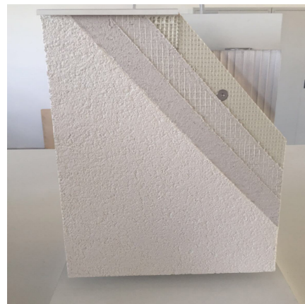
A close-up look of a mock-up to demonstrate the essential layers of a good plastering system.
