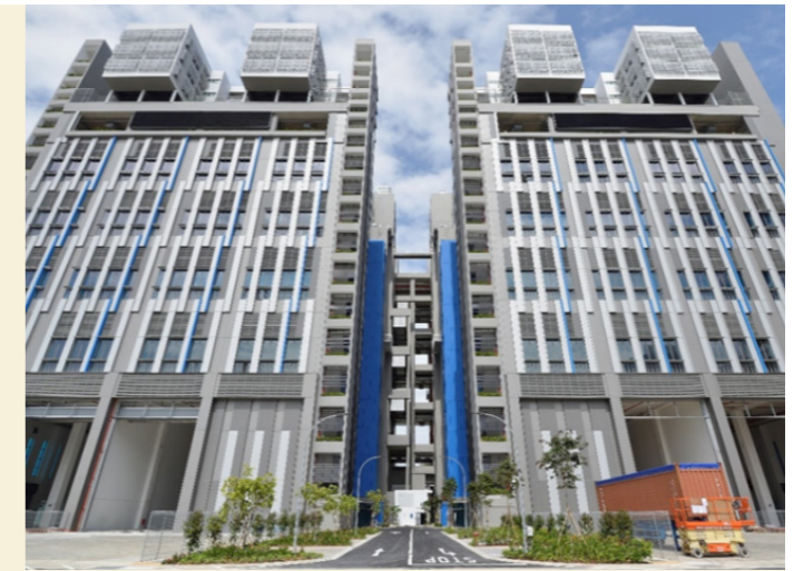
JTC Space @ Tuas was the first JTC development to adopt PPVC technology.
