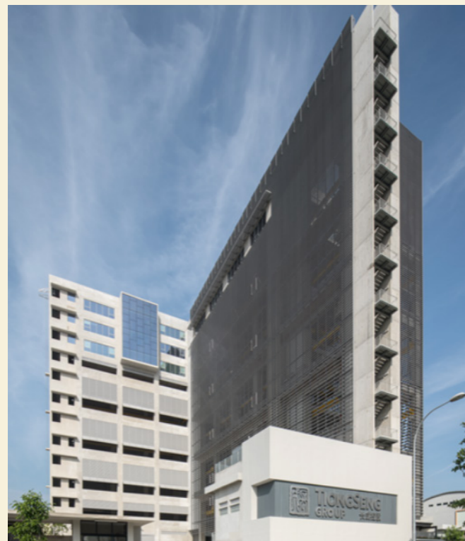
The Tiong Seng Building at 21 Fan Yoong Road.
