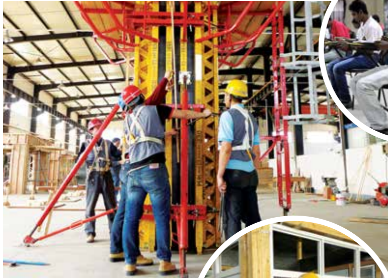
Above and left: Enhanced System Formwork Installation incorporated with Work-At-Heights Theory Test.
