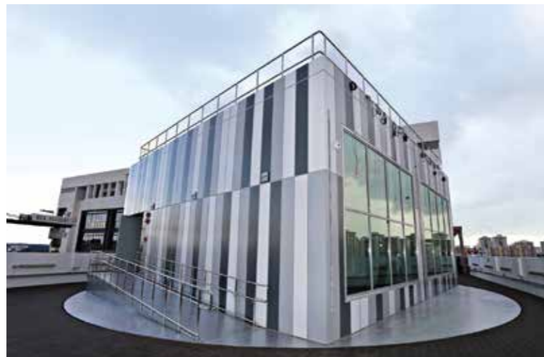
BCA SkyLab is a purpose-built, rotatable, state-of-the-art facility to test and develop energy-efficient building technologies.
