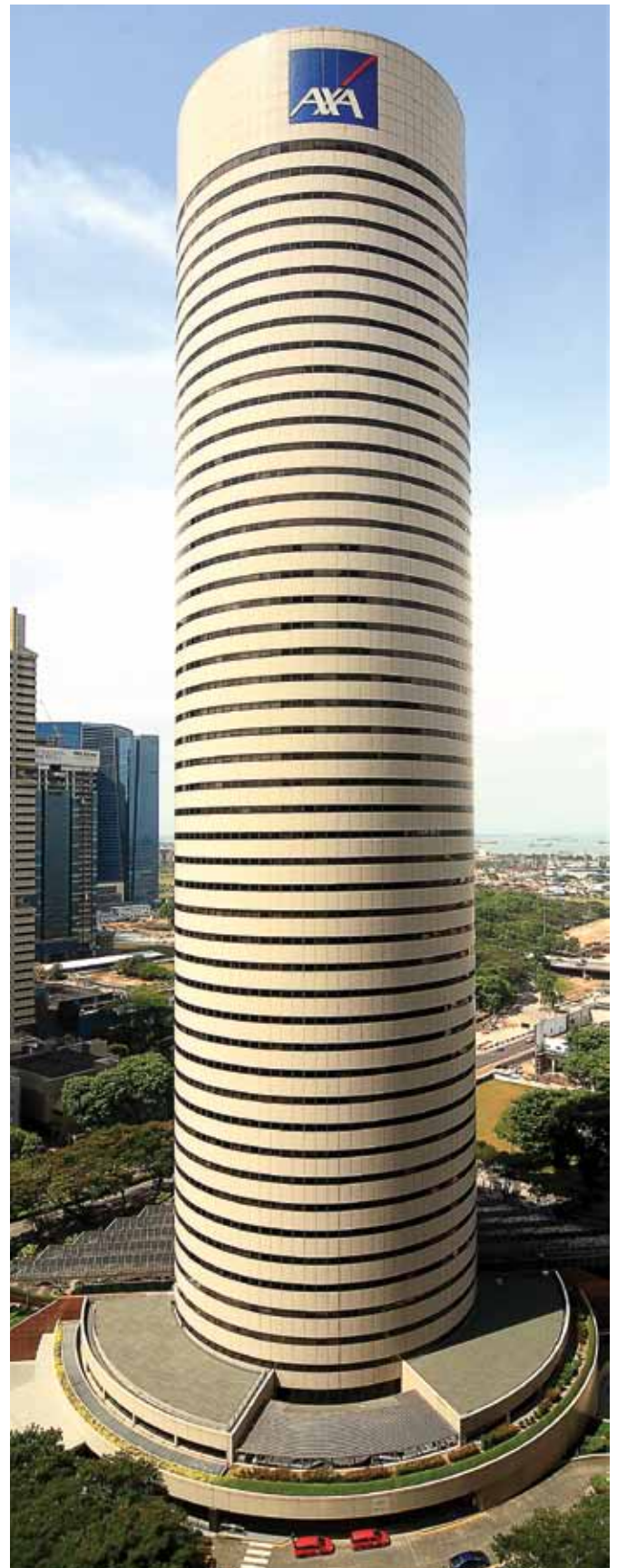
Above | The AXA building achieves energy savings of 2,047,985 kWh/year through its centralised chilled water air-conditioning system and a Building Automation System (BAS) to monitor its air-conditioning and Mechanical Ventilation System as well as other systems.
