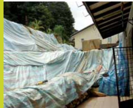
protective measures for affected slopes and houses
