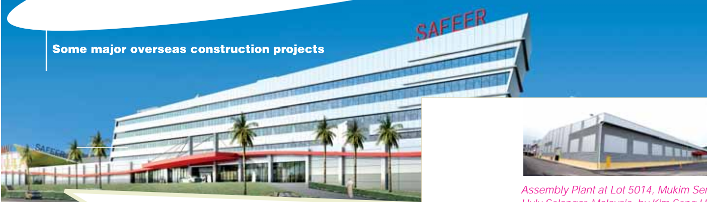
Safeer Mix Mall & Hotel Development in Fujairah, UAE, by Koon Seng Construction Pte Ltd
