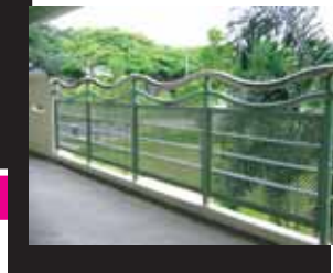
Steel railings with aluminium perforated panels
