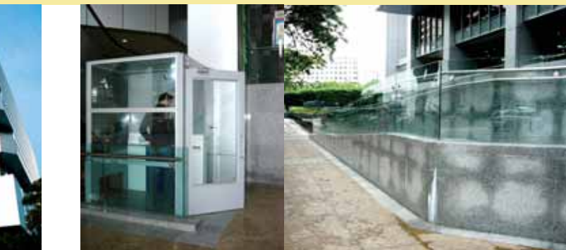
Singapore Power Building and its new accessibility features
