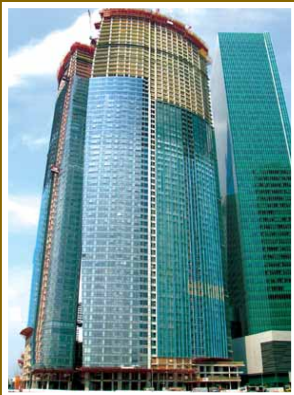
The Sail @ Marina Bay uses high strength concrete
