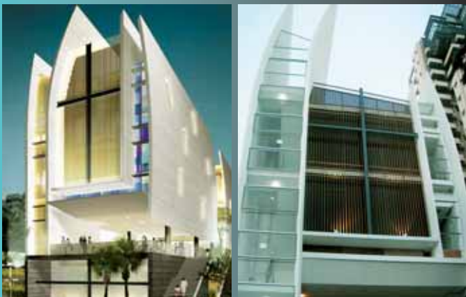
Rendered image (Left) vs as-built Revival Centre Church (Right) Images courtesy of LAUD Architects Pte Ltd
