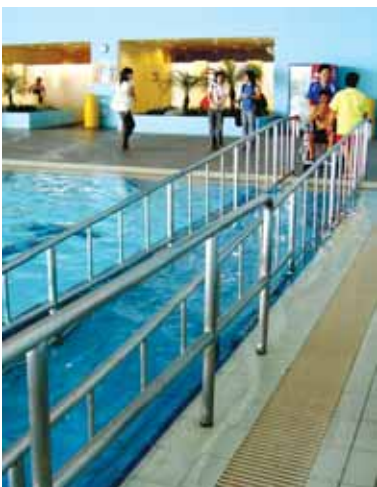
Barrier-free access into pools at Sengkang Sports & Recreation Centre, UD Award Gold winner 2009
