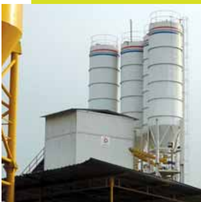
The Samwoh Ready-Mixed Concrete Plant
