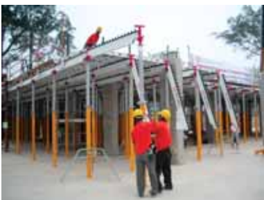
Technology Adoption: Use of Integrated System Formwork
