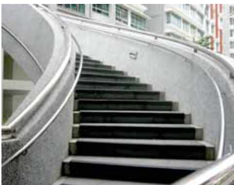
Two sets of handrails at different heights for people of different statures at Sengkang Aspella, UD Award Bronze winner 2009
