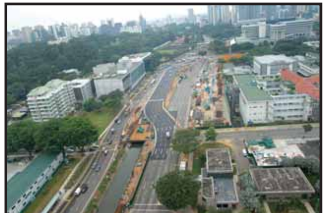
Temporary public vehicular deck over Rochor Canal
