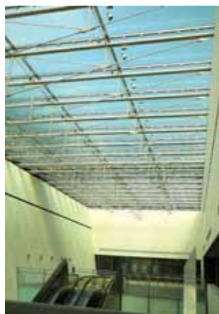
Construction and Completion of Dhoby Ghaut, Bras Basah, Esplanade and Promenade Stations and Tunnels – Circle Line Stage 1 C825
