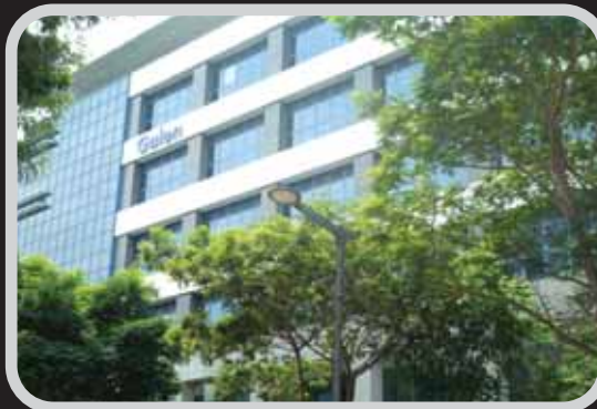
The Galen (Non-Residential Existing Buildings)
