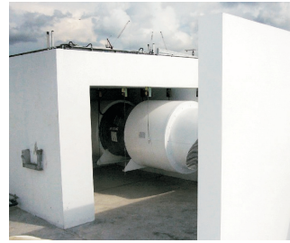
View of RC tunnel wall used to protect blast hatch
