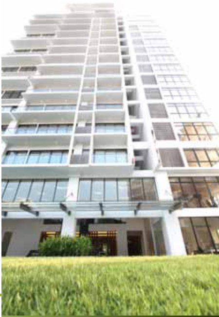
Ken Bangsar, Malaysia (Residential New Buildings) Gold Plus
