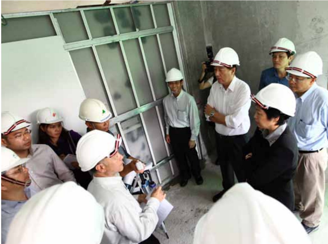
Left | The first stop was the mock up unit. The delegation was briefed on the buildable features of drywall and shown the different stages of installation. They were also briefed on how these features reduced the amount of wet trades on site before they viewed the final PBU product.
