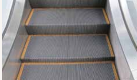
Left | Close-up of an escalator with no deflector devices. Bottom Left | Close-up of brushes.
