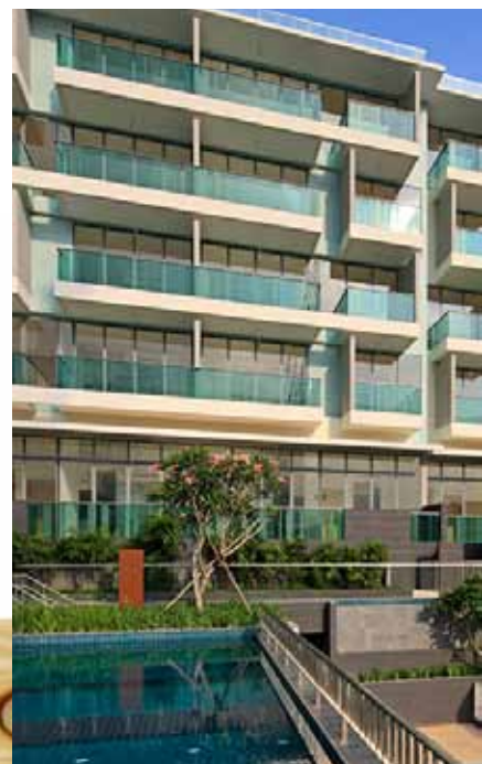
Right | Shelford Suites is one of Tiong Seng’s projects to have achieved a STAR rating under the new Tiered Rating for Quality Mark.
