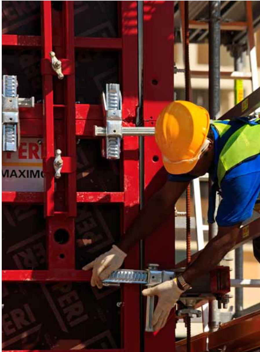
Above | Utilizing advanced formwork systems.
