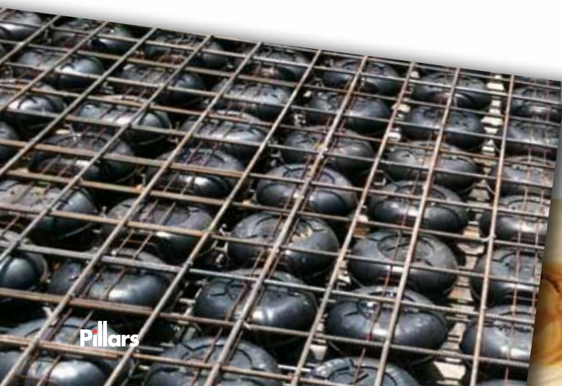
Left | Cobiax is an internationally-patented construction method which reduces carbon emissions and improves structural efficiencies.
