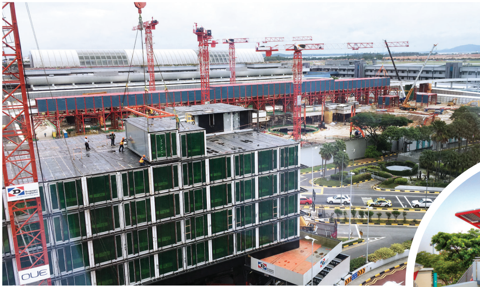
Left: With the introduction of Prefabricated Prefinished Volumetric Construction (PPVC), there will be less noise and dust at construction sites as more activities are done off-site.
