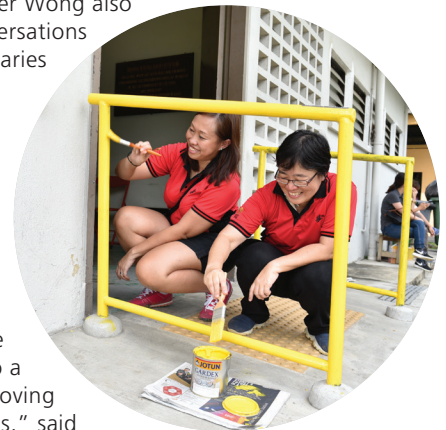
Below: BCA volunteers repainting the railings at SAVH.
