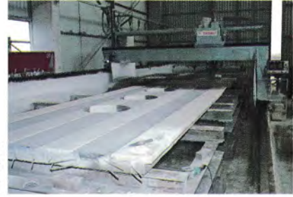
Machine polishing a two-tone precast concrete panel
