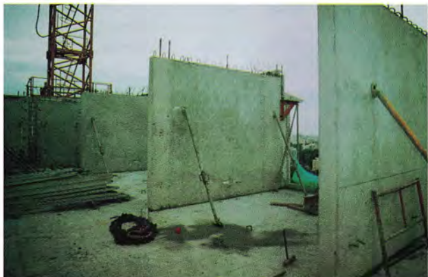
Temporary support for precast wall panel
