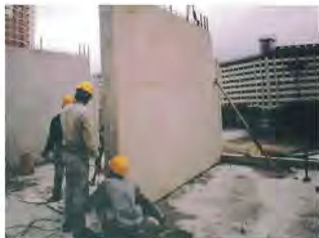
Precast projects use fewer workers, cutting down labour cost
