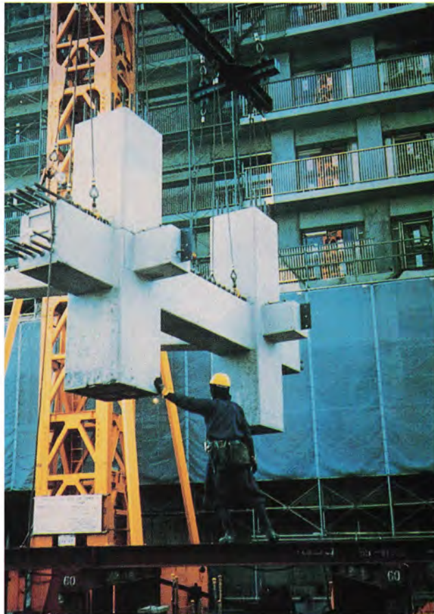
Erection of precast H-shaped unit
