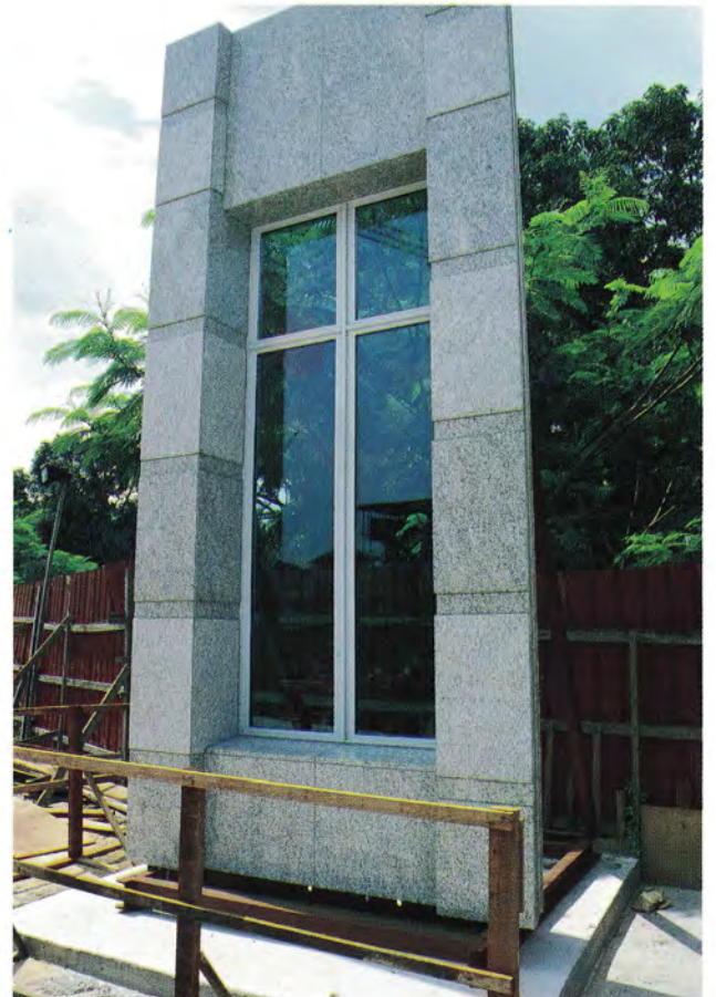
Ministry of Home Affairs Complex: Granite in honed and polished finish in precast facade. The full prototype panel incorporates aluminium frame to achieve weather-tight joints
