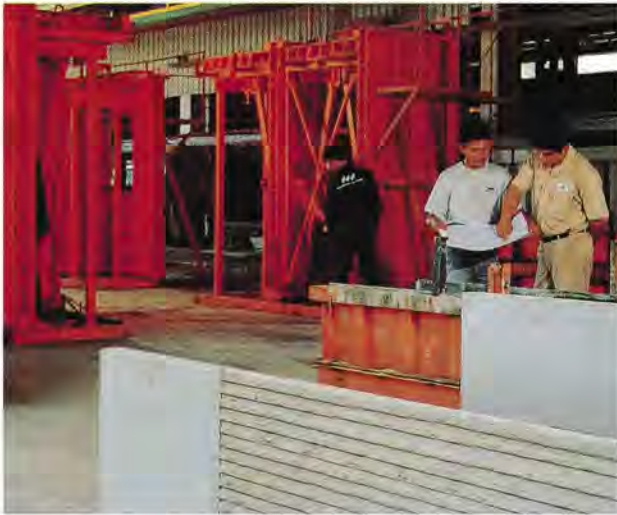
Efficient production schedule through good co-ordination
