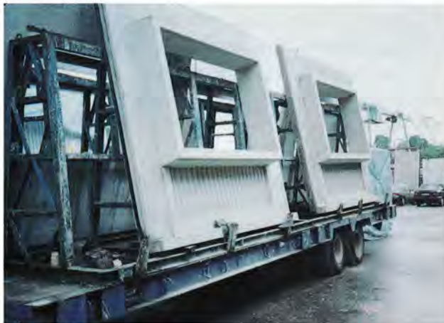
Wall panels transported by a low trailer
