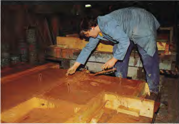
By using largest panel as a master mould concept, different section of the panel is being cast or blocked off
