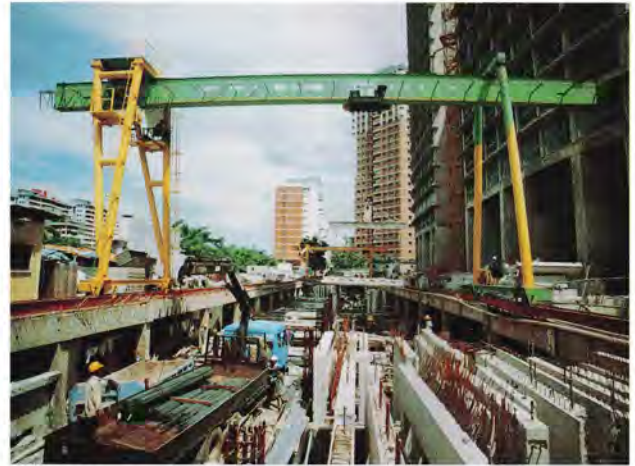
Site casting and handling
