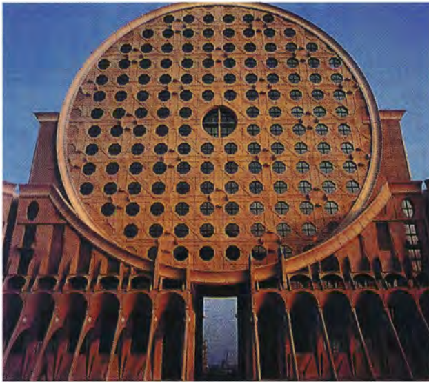
Public housing Les Arènes De Picasso In Paris: Fully-precast standardised architectural facade Architect: Manolo Nunez Yanowsky Source: Omnium Technique OTH
