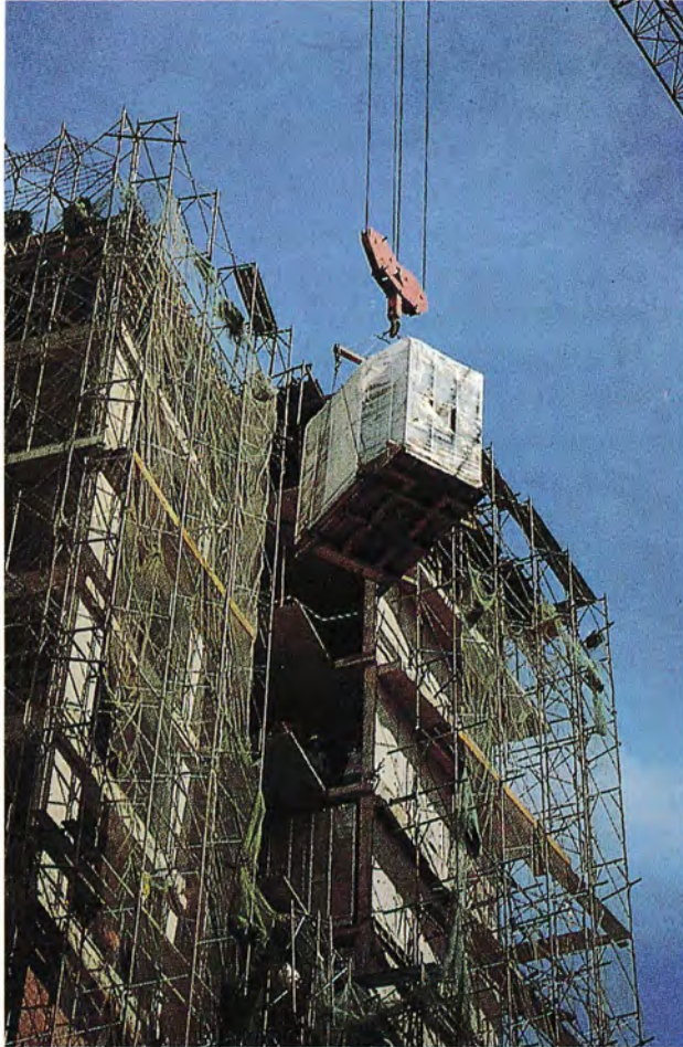
Hoisting of prefabricated toilet unit
