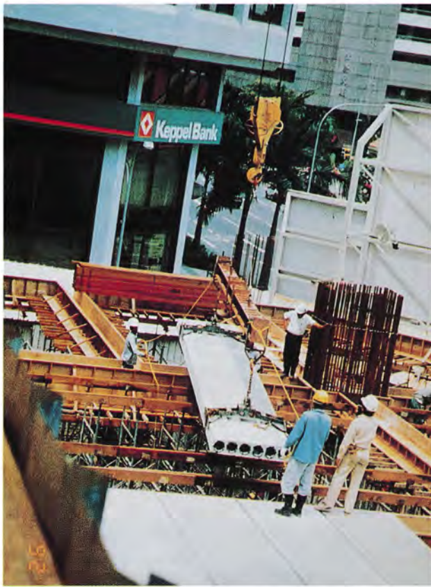
Installing hollow core floor
