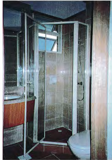
Completed interior of Trellis Towers prefabricated bathroom
