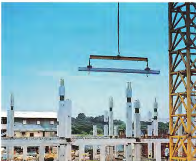
Selection of type and capacity of crane will depend on size and weight of precast component
