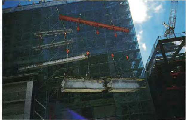
Lifting of precast panel
