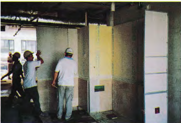
Prefabricated finished walls separately lifted and assembled at location
