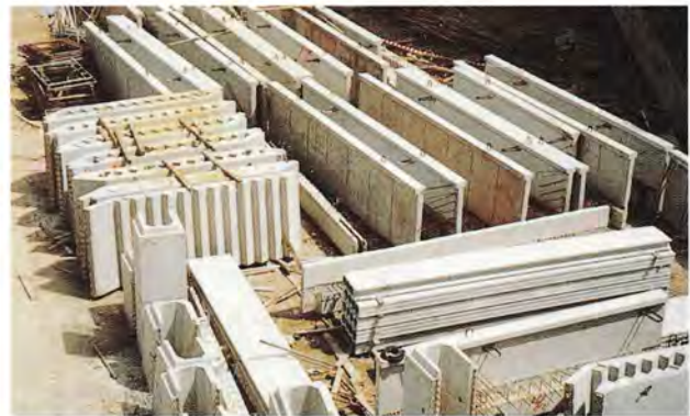
Storage of precast components on site requires careful planning
