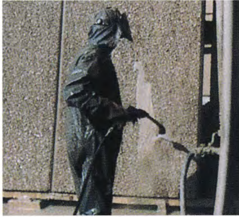
Sand blasting to precast concrete surface
