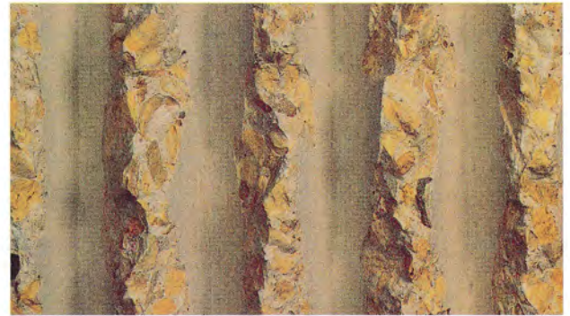
Rope and hammered nib textured surface
