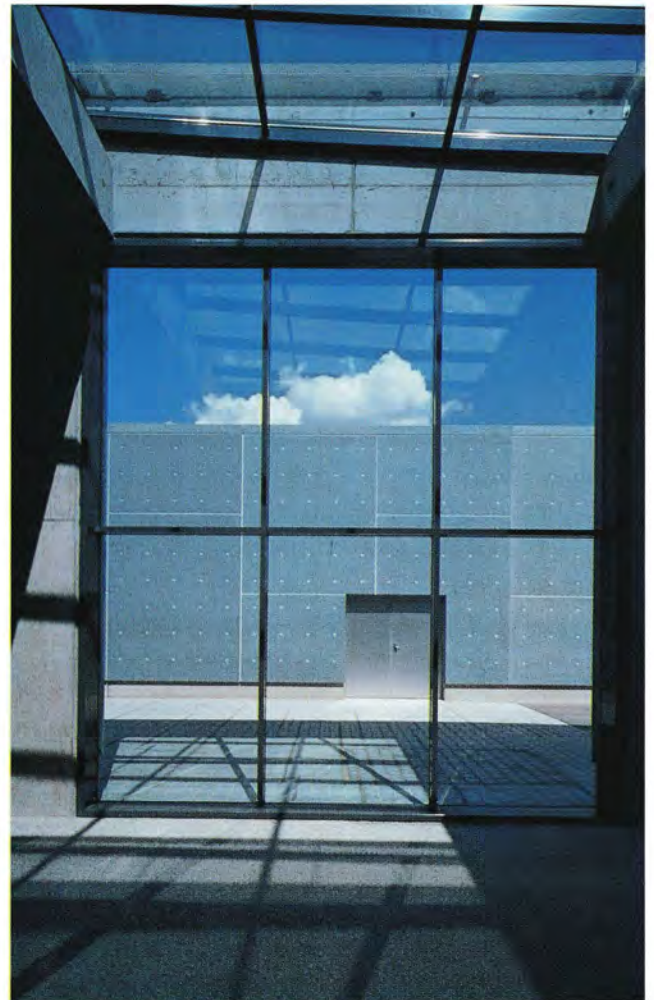
Blue coloured pigment concrete wall with a surface water repellent treatment to protect exposed surface from water and atmospheric pollution. Usine des eaux de joinville Le Pont Architect: Jacques Ferrier
