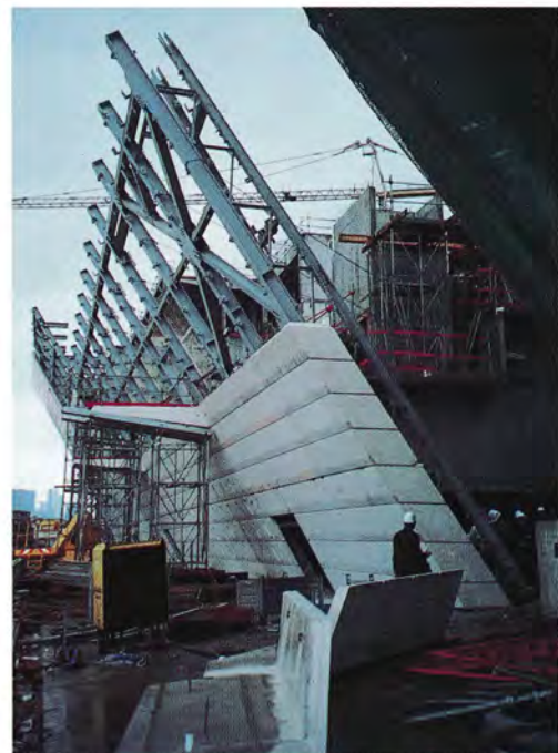
Precast polished concrete facade on steel structure: Palaise De congress Architect: Christian de Portzamparc, Paris
