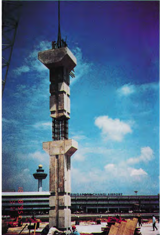
Precast column: Changi Airport Terminal 2
