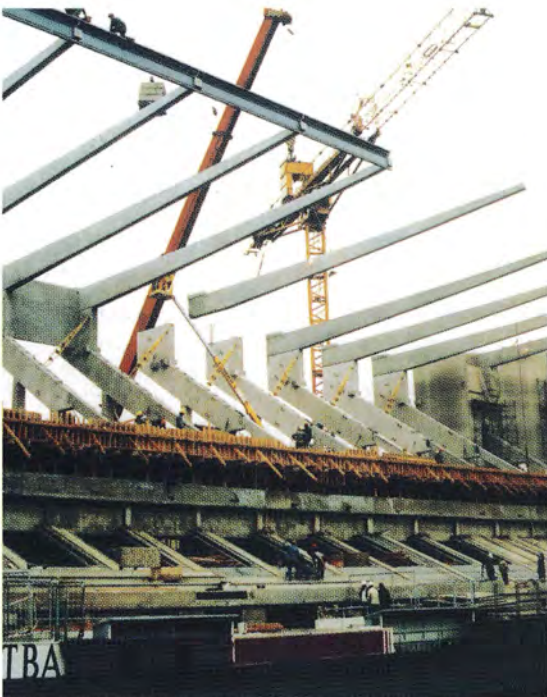
Precast and prestressed roof beams: Anderlecht Stadium in Brussels
