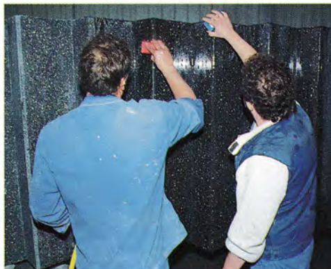
Final hand polishing to a polished concrete staircase
