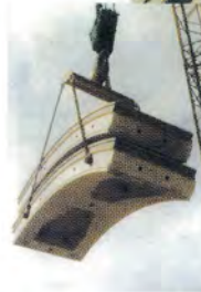
Precast segmental linings to underground Mass Rapid Transit System in Antwerp
