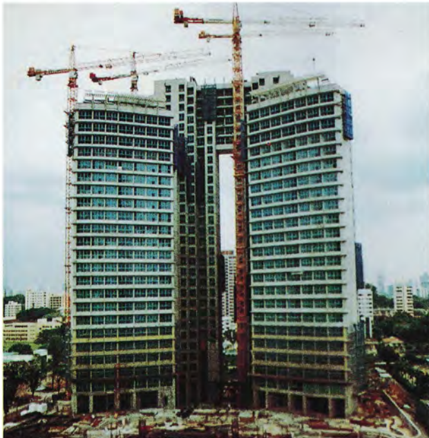
Trellis Towers: Precast load-bearing walls are adopted for third storey onwards
