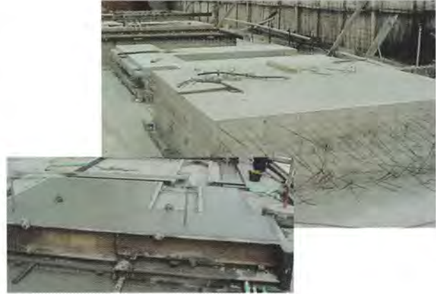
Stack casting of wall panels reduces formwork and storage costs
