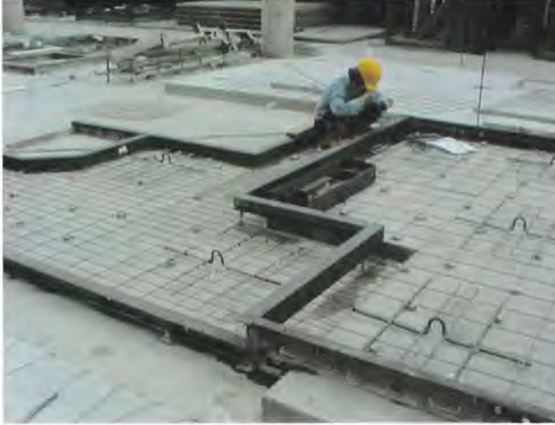
The new trend: On-site precasting
