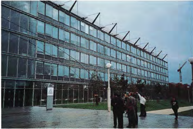
Exterior view of The National School of Civil Engineering and Geographic Sciences, Paris
