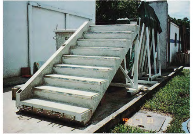
Precast concrete staircase
