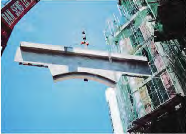
Lifting precast components
