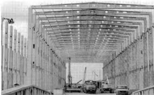
Single storey industrial building
