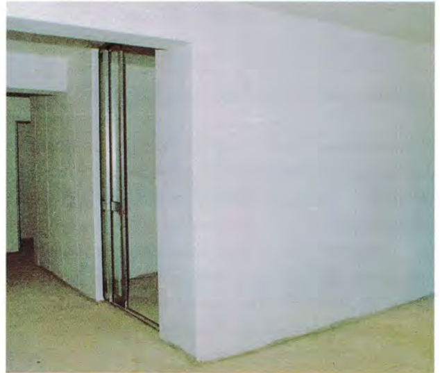
Finished precast internal wall
