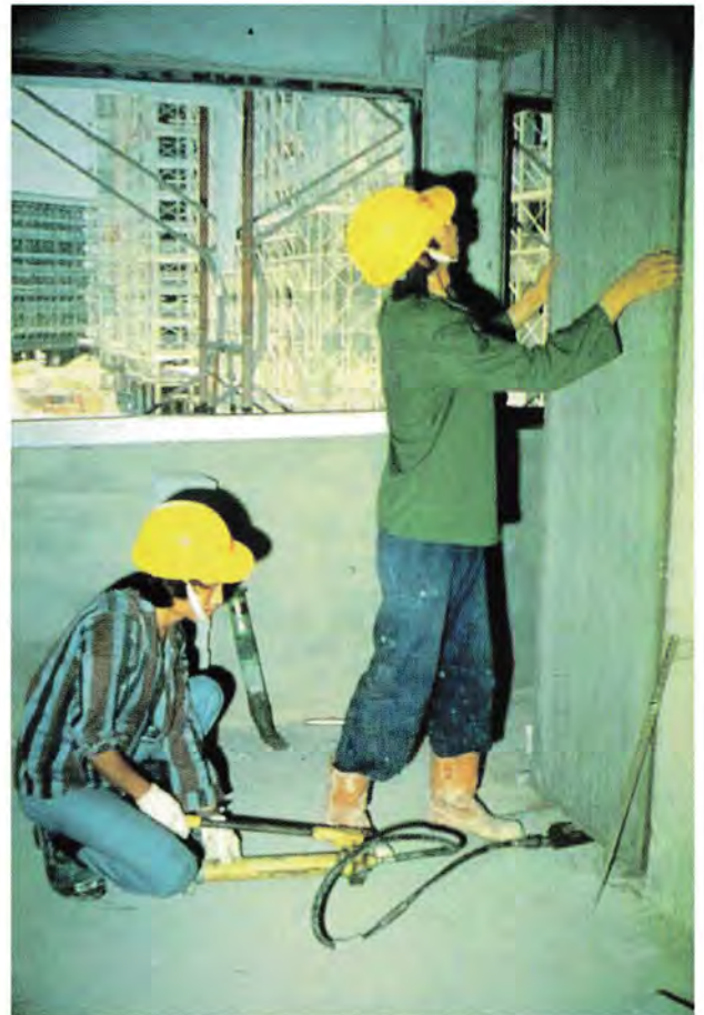
Installation of precast concrete lightweight panel
