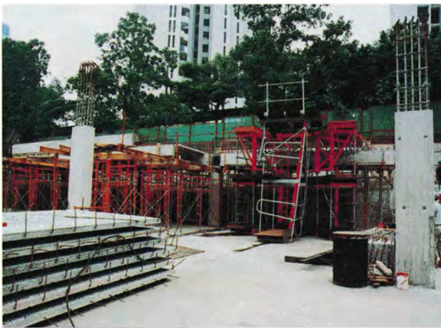
Hazel Park: (Above) Lifting the room-size precast half-slab (Below) Precast half-slabs ready for installing over precast beams
