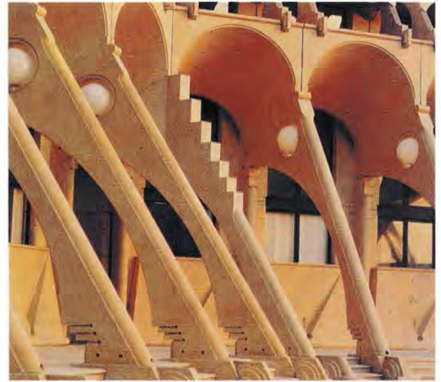
Public housing Les Arènes De Picasso In Paris: Fully-precast standardised architectural facade Architect: Manolo Nunez Yanowsky Source: Omnium Technique OTH
