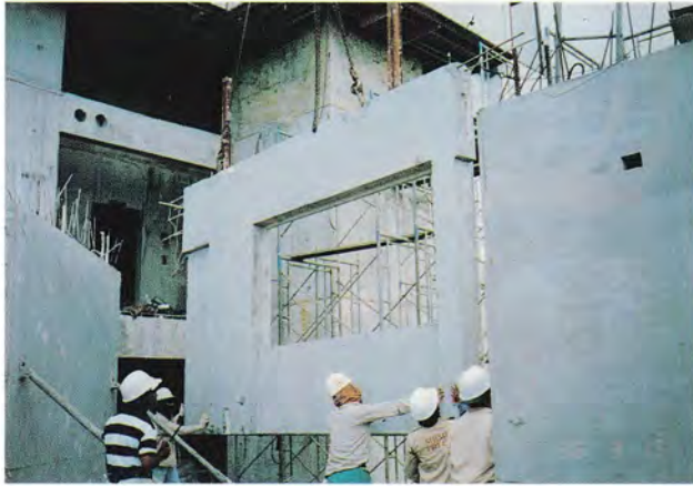
Erection of precast wall panel
