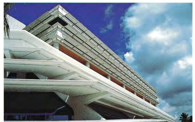
Precast roofs to carpark building: KK Women and Children Hospital Singapore
