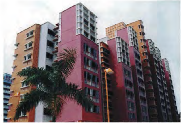
Public housing at Yishun Street 20: Modular co-ordinated design
