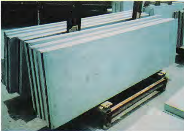
Stacking of precast internal wall panels
