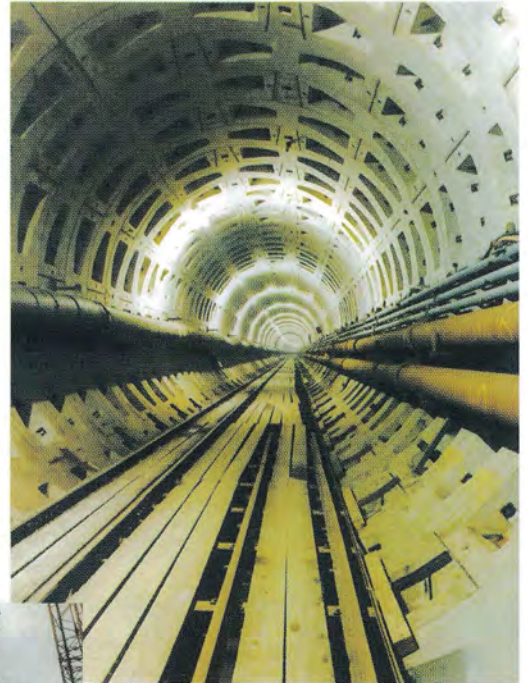
Precast segmental linings to underground Mass Rapid Transit System in Antwerp
