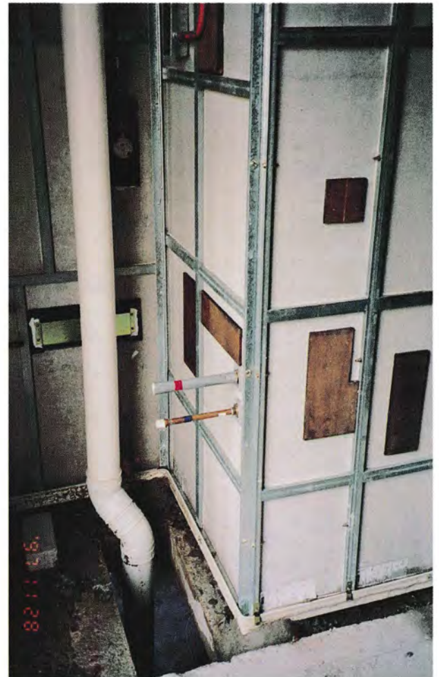
Connections to soil stack
