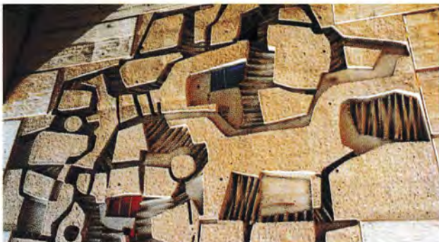
Sculptured precast wall reflects the plasticity of concrete
