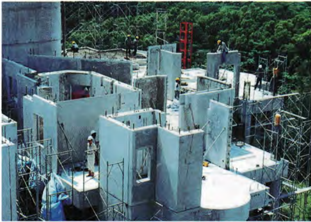
The Bayshore Condominium: (Above) Load bearing precast wall (Below) Completed building
