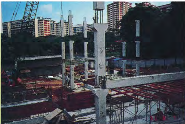
Multi-tiered precast columns
