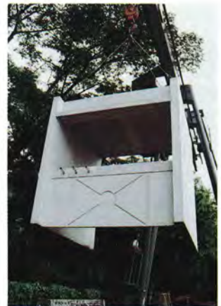
Precast service balcony
