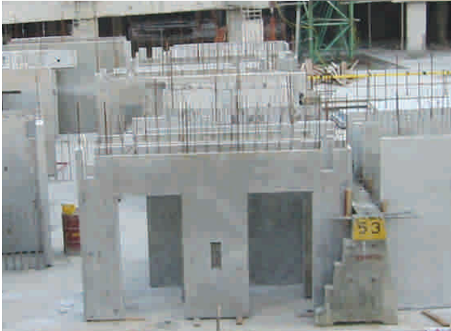
Fig. 1.26 – Precast lift lobby wall can be used for better finishes
