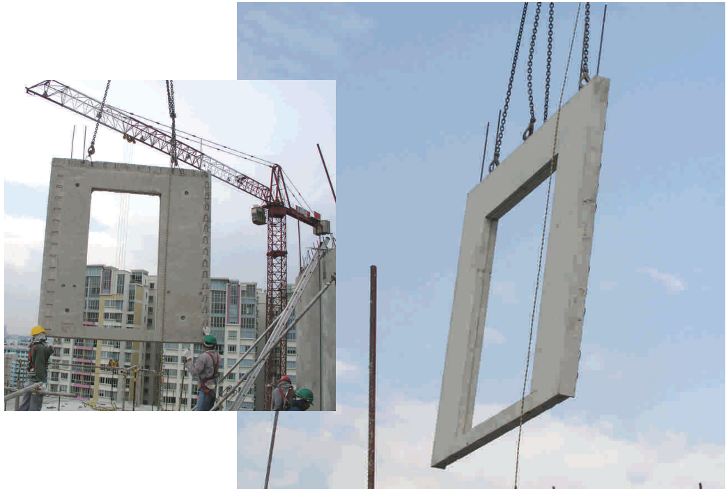
Fig. 1.11 – Hoisting of precast panels is essential for erection
