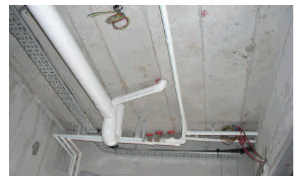
Fig. 3.4 – With add-on ceilings, all services can be concealed within the ceiling space after installation
