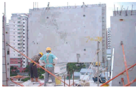
Fig. 6.9 – Lowering of precast wall panel during installation
