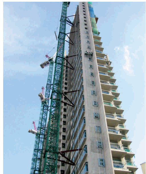
Fig. 6.47 – Two cranes for each block
