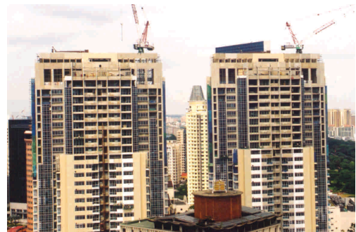
Fig. 6.33 – Newton.GEMS under construction
