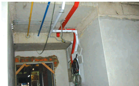
Fig. 3.4 – With add-on ceilings, all services can be concealed within the ceiling space after installation
