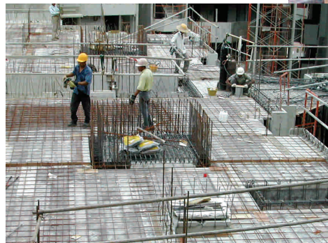
Fig. 6.10 – Preparation for casting of in-situ flat plate
