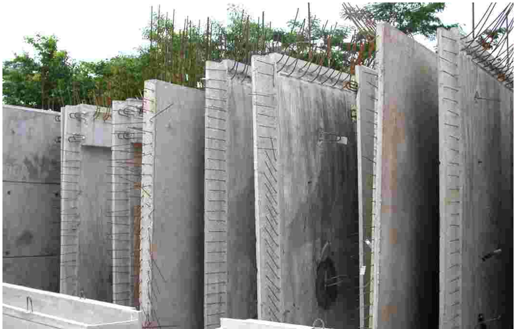
Fig. 4.4 – Secure vertical panels on racks at appropriate spacing
