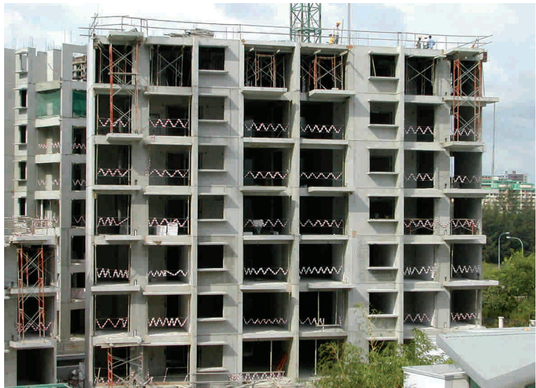
Fig. 6.4 – With proper jointing, the need for external scaffolding system was eliminated
