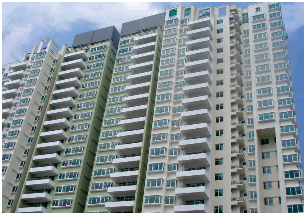
Fig. 6.30 – Closer view of the building completed
