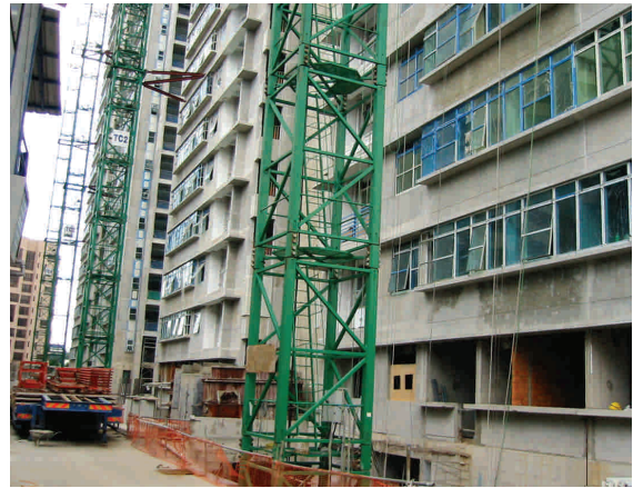
Fig. 6.37 – Limited site access for panel delivery
