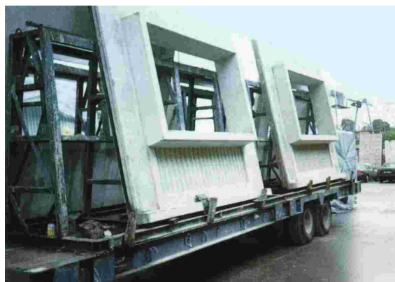
Fig. 4.2 – Wall panels transported by a low trailer
