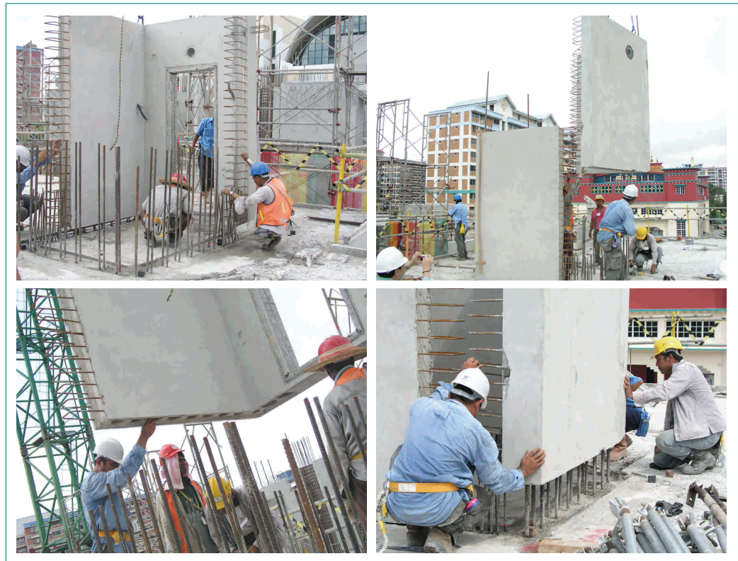
Fig. 1.31 – Installation of precast household shelter in 2 'L-shaped' panels
