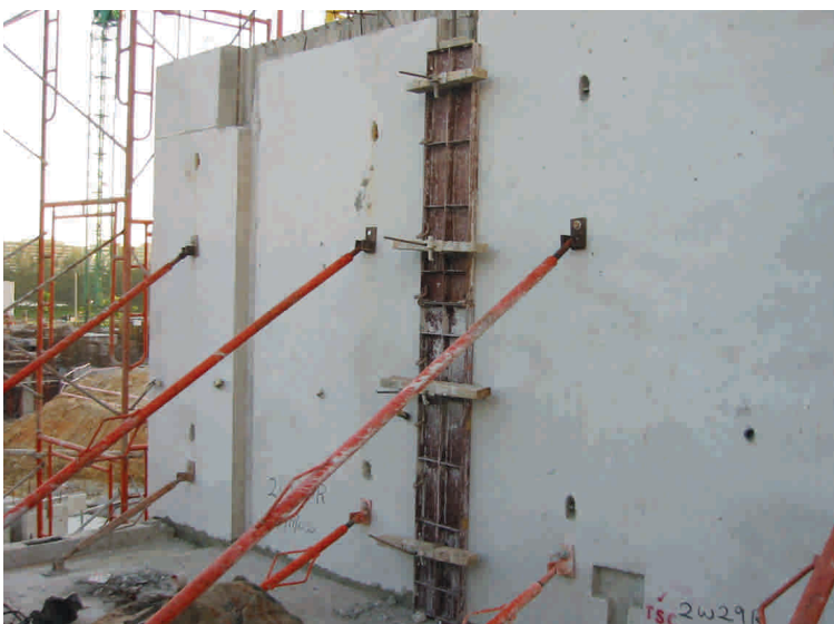
Fig. 1.24 – Casting of in-situ vertical joints
