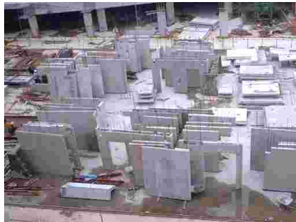
Fig. 4.3 – Ground level of storage area should be relatively level and firm
