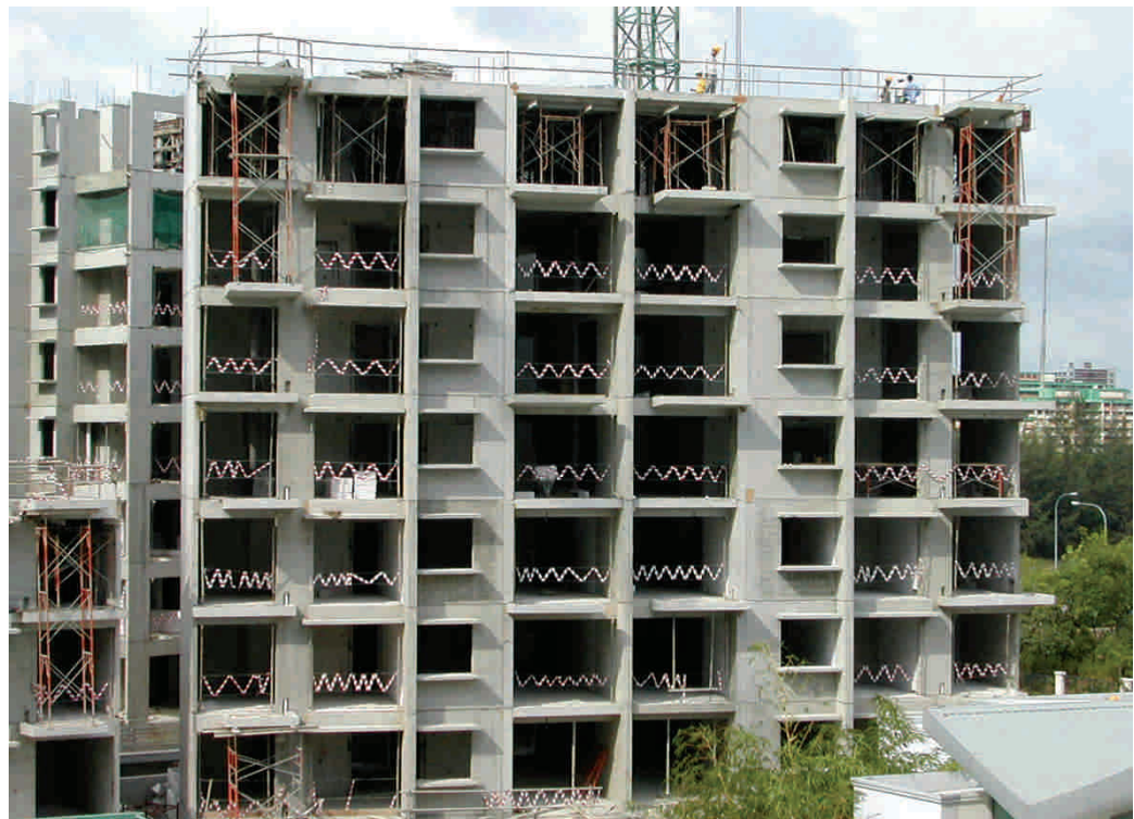
Fig. 6.4 – With proper jointing, the need for external scaffolding system was eliminated
