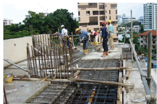
Fig. 6.49 – Casting of pour strip after installation of precast floor slab
