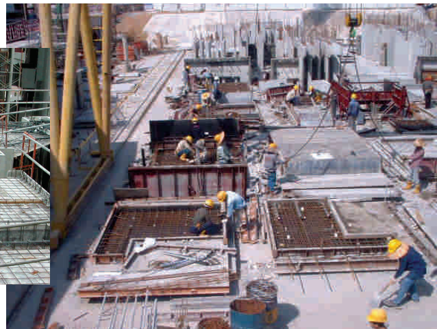
Fig. 6.11 – On-site precasting for simpler components
