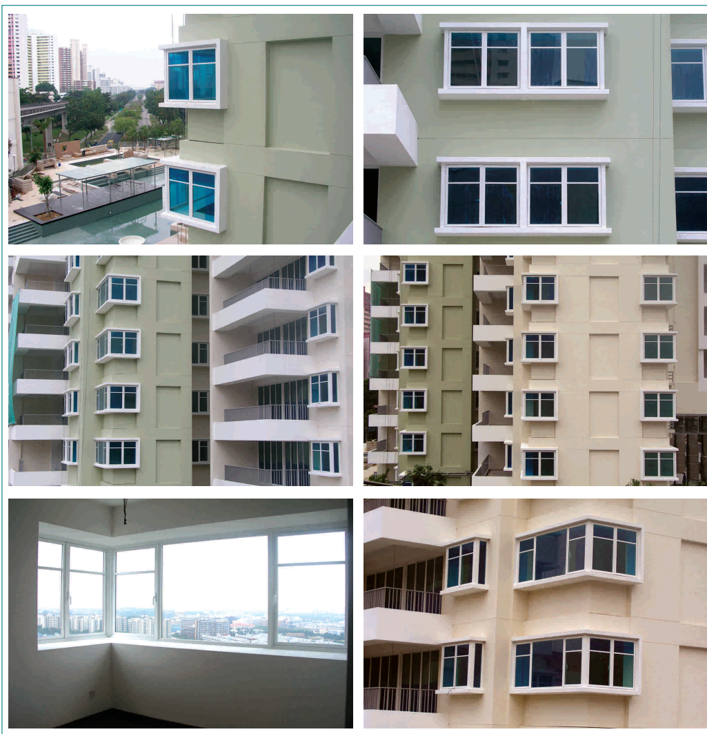
Fig. 6.31 – Better wall finishes can be achieved using precast façades comprising window wall units and bay windows
