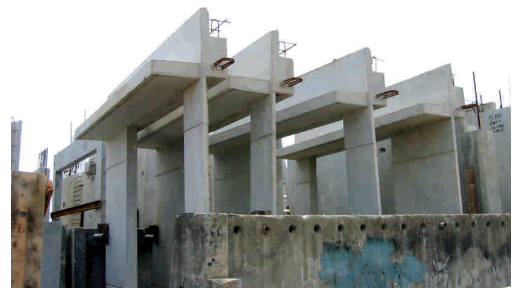
Fig. 6.43 – Non load-bearing window wall integrated with beam to form an enclosed window panel
