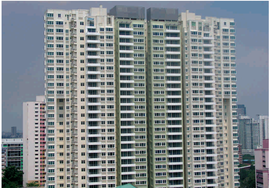
Fig. 6.29 – Overview of the building envelope using non load-bearing precast façades
