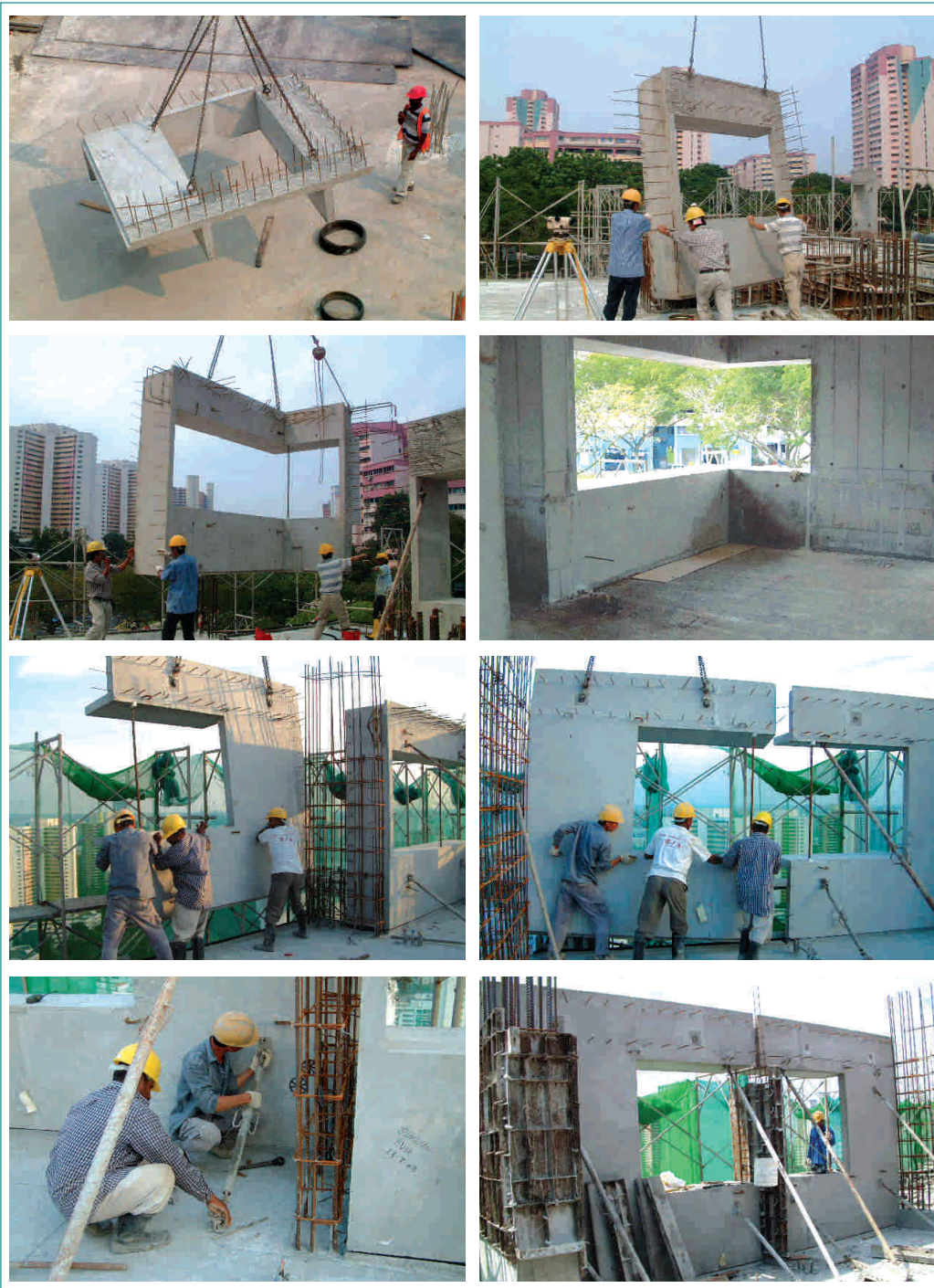
Fig. 6.28 – Installation of different non load-bearing precast façade wall elements
