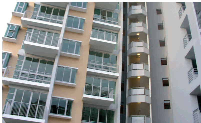
Fig. 6.16 – Use of precast staircase and landing
