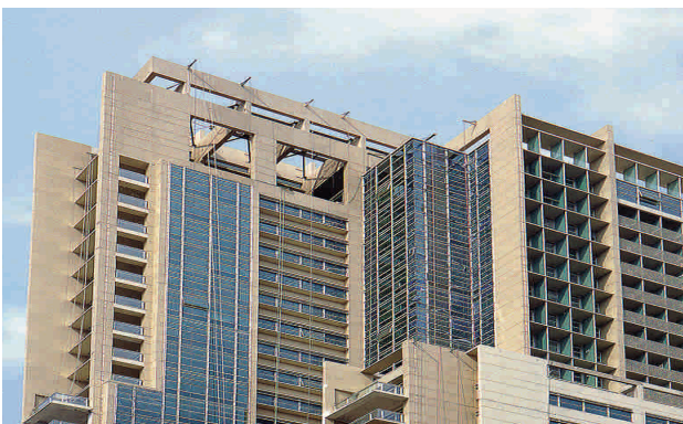
Fig. 6.46 – Photo showing part of the crown structure at about 15 m above the building roof level
