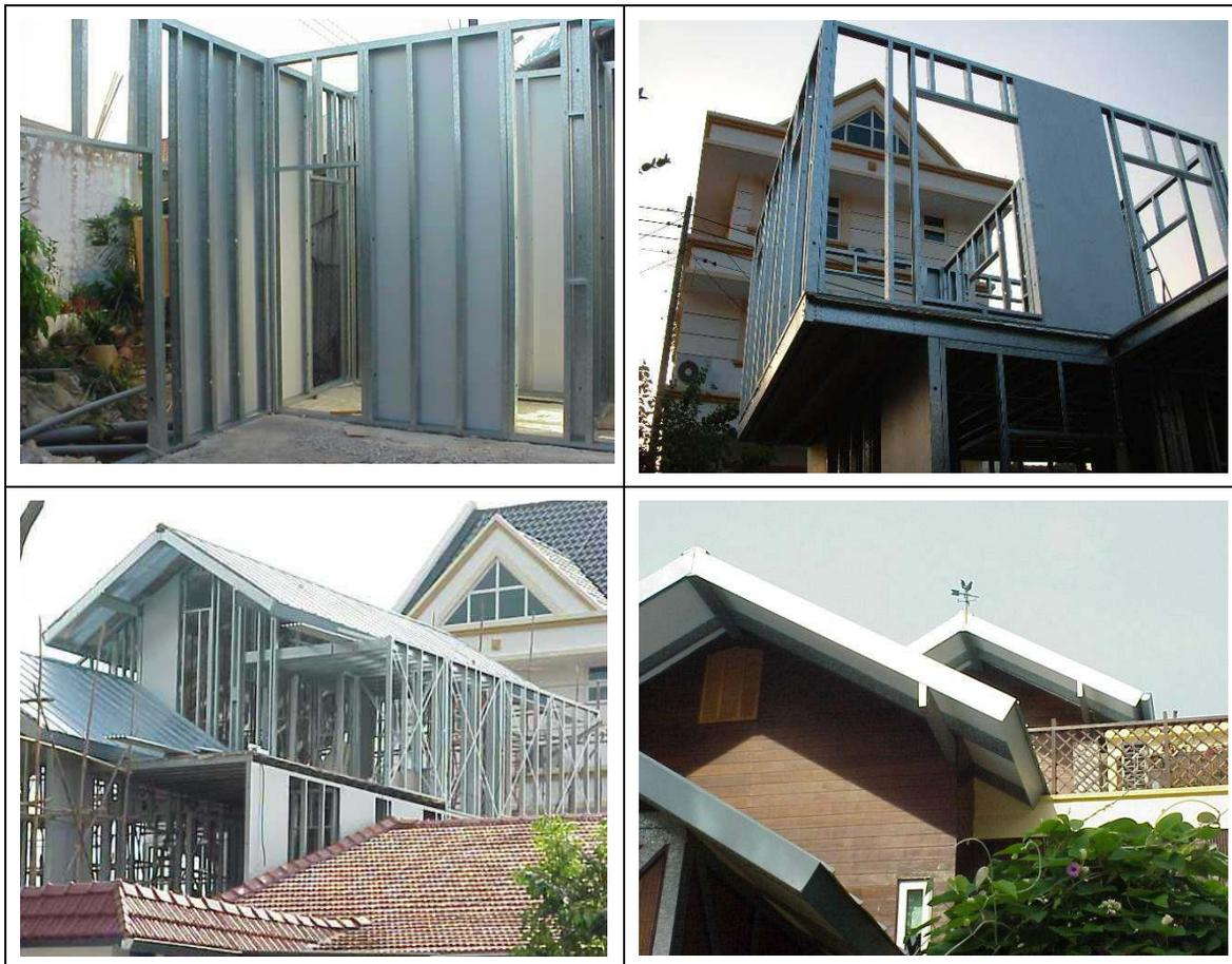
Figure 10.1 Construction of lightgauge steel frame
