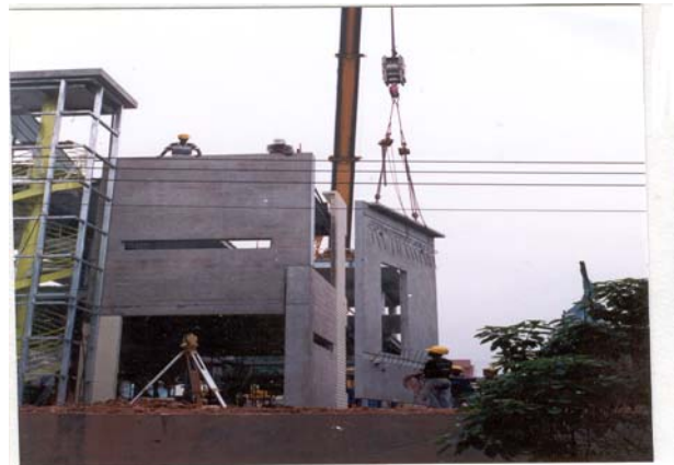
Figure 2.2 Hoisting of precast facade
