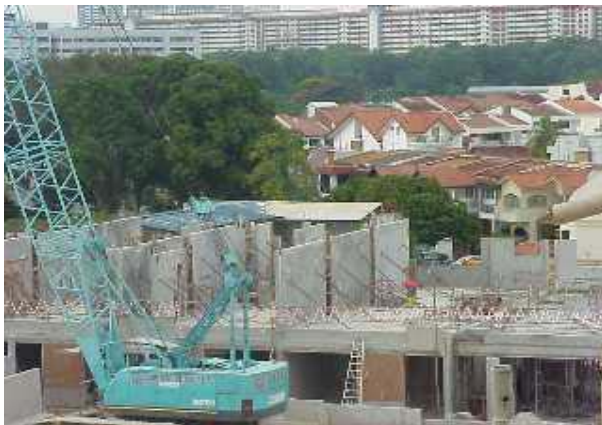
Figure 2.1 Use of 50-tonne crane for hoisting
