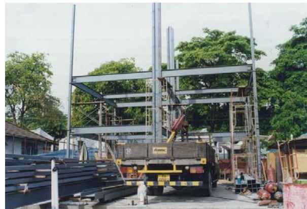
Figure 2.4 Use of lorry crane for lifting of steel elements
