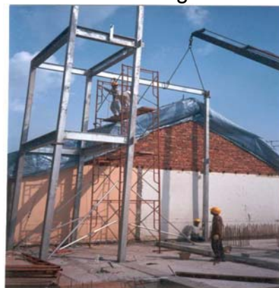
Figure 2.3 Assembly of steel elements in position
