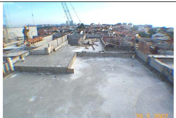
Figure 4.6 Concreting to topping
