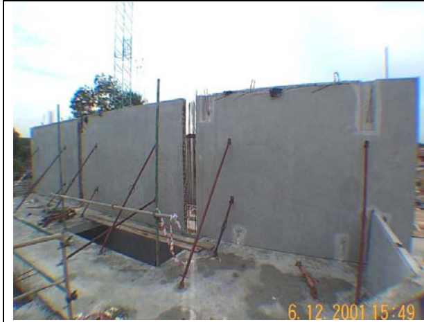
Figure 4.1 Precast walls are propped before casting of joints – proper planning is required for perfect alignment
