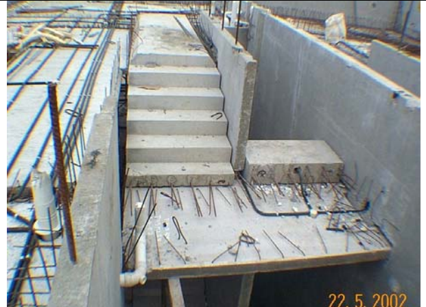
Figure 4.4 Preparation for casting of landing slab to precast staircase
