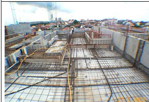
Figure 4.5 Preparation of welded mesh and services for cast in-situ topping
