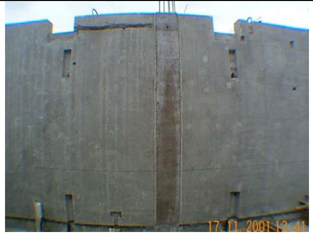
Figure 4.2 The pour strip between 2 pieces of precast walls are cast
