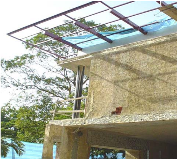
Figure 6.1 Construction of circular steel hollow section with cast in-situ flat plate
