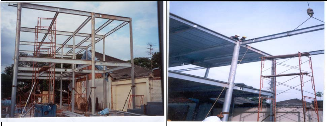
Figure 8.2 Bolted connection for column to beam with laying of metal decking for second storey and roof
