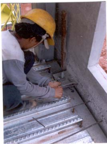
Figure 8.4 Fastening of connection
