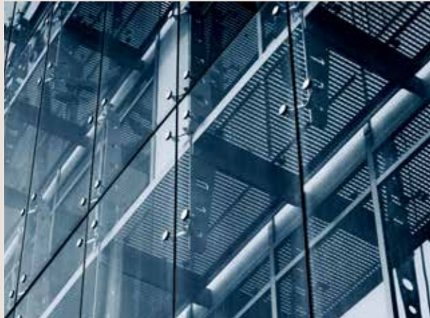
Figure 25: Example of a point supported curtain wall
