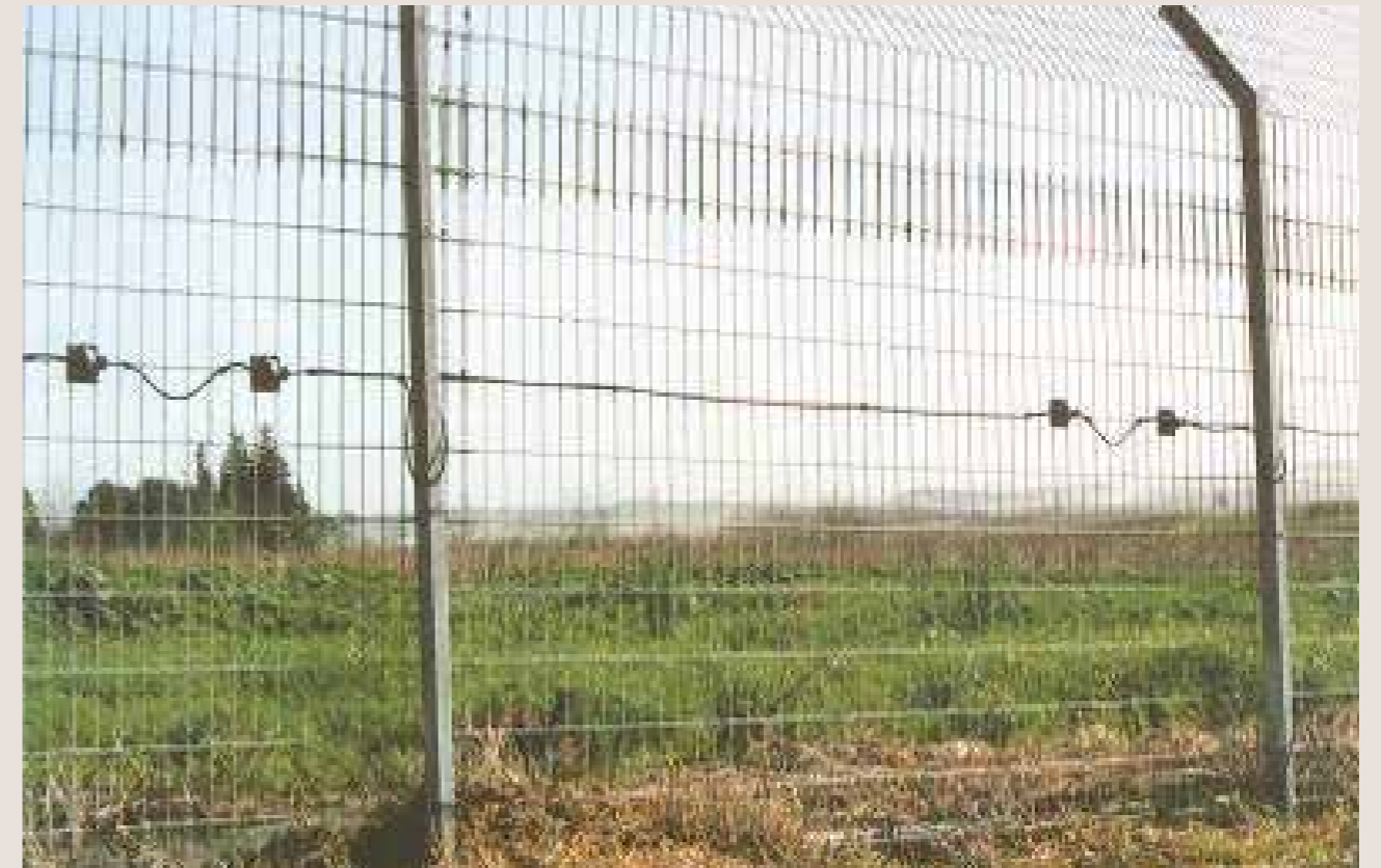
Figure 9: A welded mesh fence with sensor line
