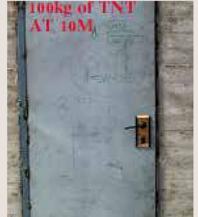
Figure 43: Blast resistant door after a 100kg explosion at 10m
