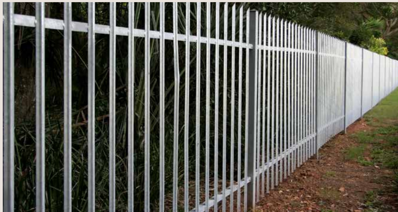
Figure 11: A typical steel profile fence
