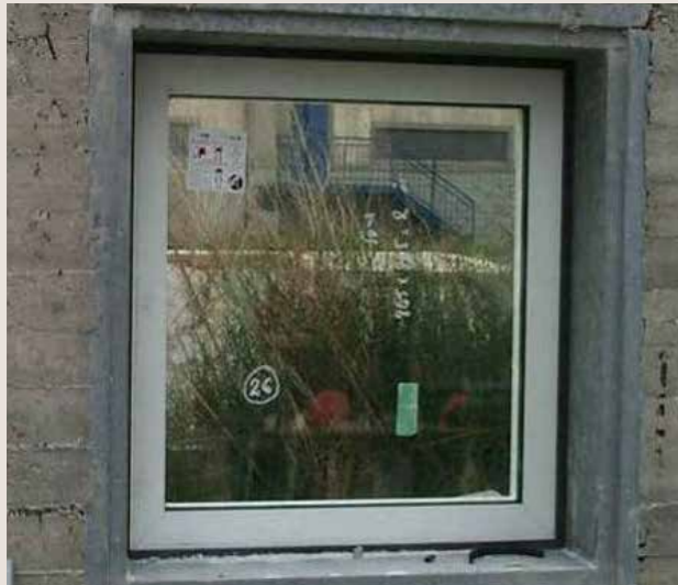
Figure 36: Window before forced entry testing
