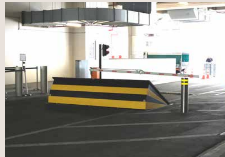
Figure 2: A crash-rated wedge vehicle security barrier.
