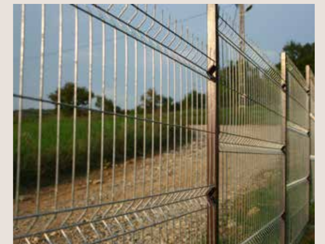
Figure 10: A welded mesh fence
