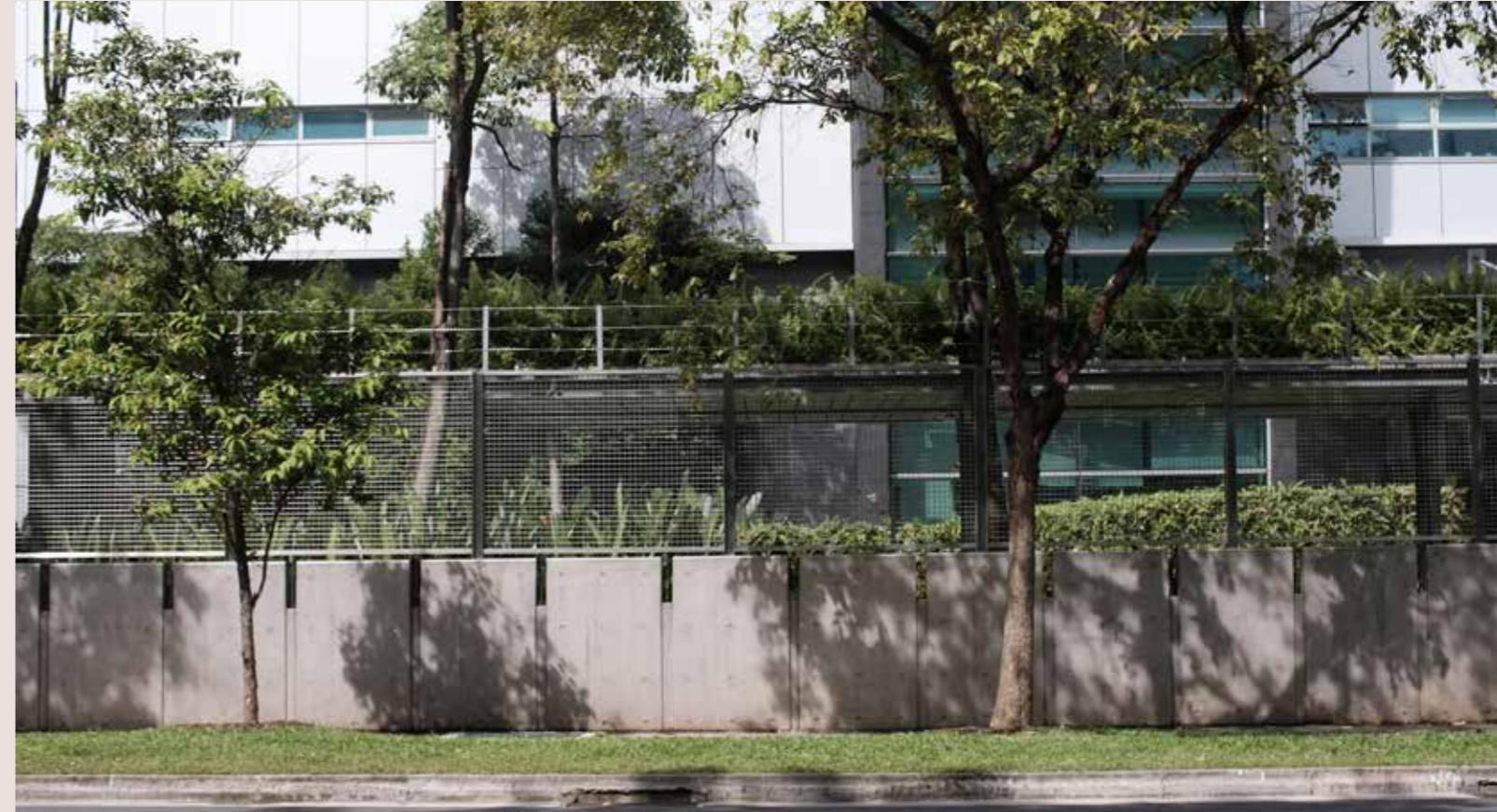
Figure 8: Example of an anti-intrusion perimeter line.
