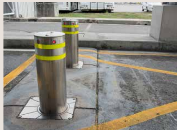
Figure 14: Retractable anti-ramming bollards
