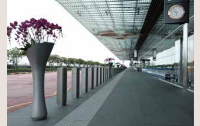
Figure 3: Bollard line with a mix of steel bollard covers and decorative bollard covers.
