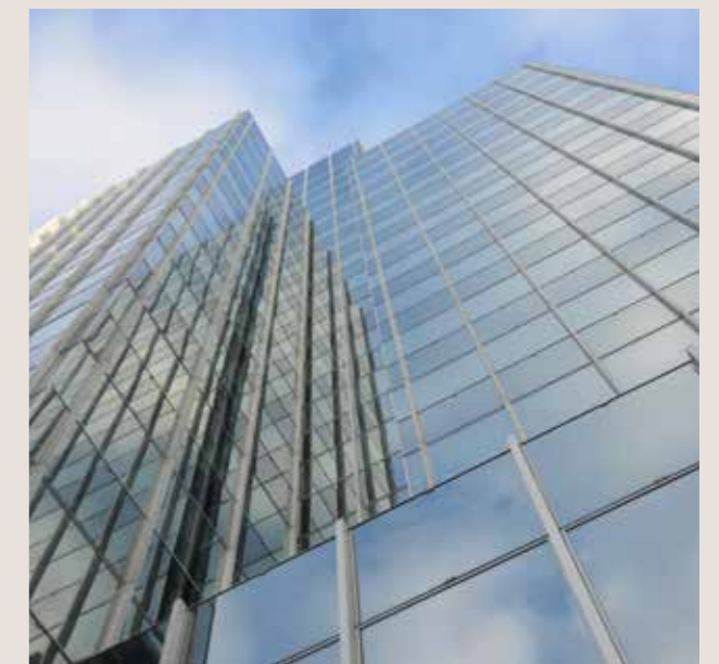
Figure 24: Example of fully framed curtain wall
