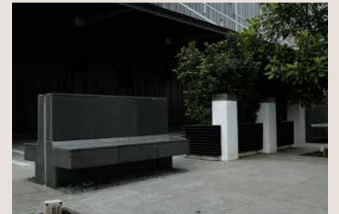
Figure 4: Bollards integrated into street furniture.
