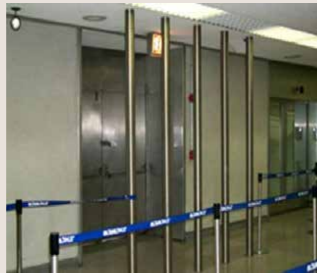
Figure 44: Steel bars used as a catcher for the doors
