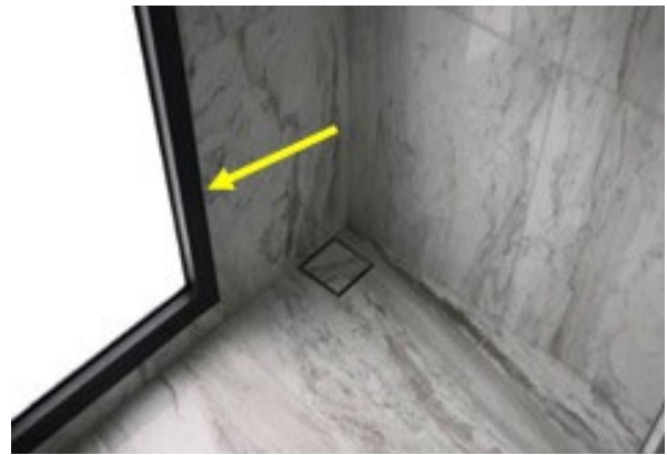
Window frame flush with wall finish surface
