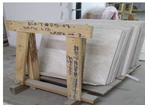
Stones stacked after dry lay
