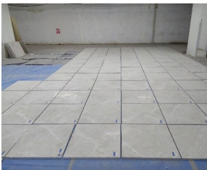
Dry lay at site
