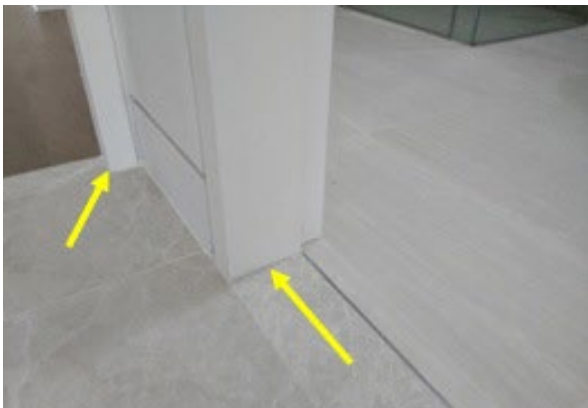
Joint at door frame covered with sealant
