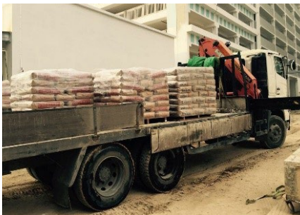
Transporting materials to site
