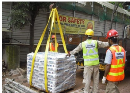
Offloading materials from truck
