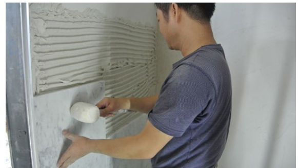
Tapping on stone for uniformity
