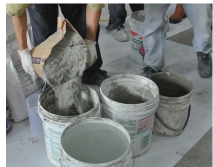
Adding powdered polymer into container
