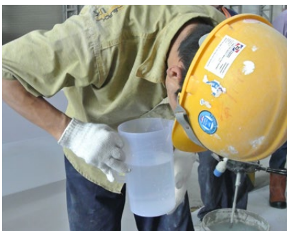
Amount of water in accordance to manufacturer's specs
