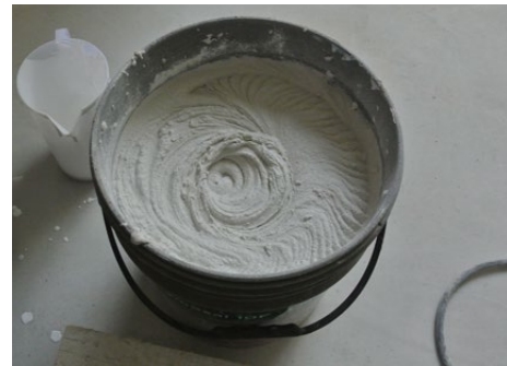
Adhesive mix ready for use
