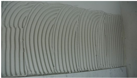
Adhesive fully trowelled
