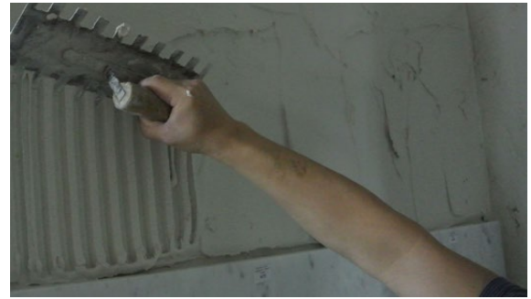
Trowelling adhesive with notched-trowel
