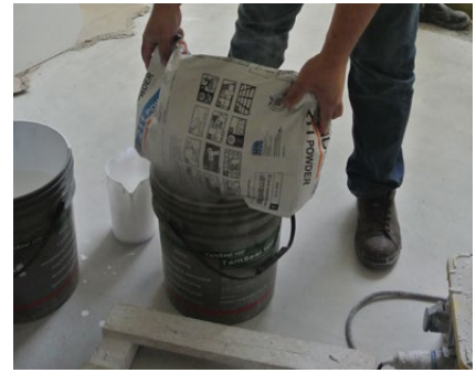
Adding powdered polymer (component 2) into the container
