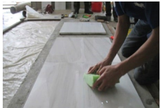
Cleaning surplus with sponge after grout had set
