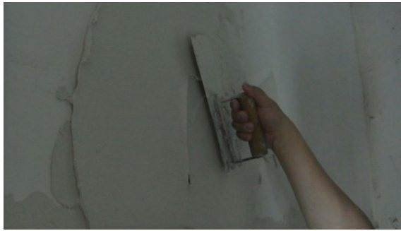
Spreading adhesive with flat side of trowel
