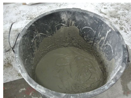
Adhesive mix ready for use
