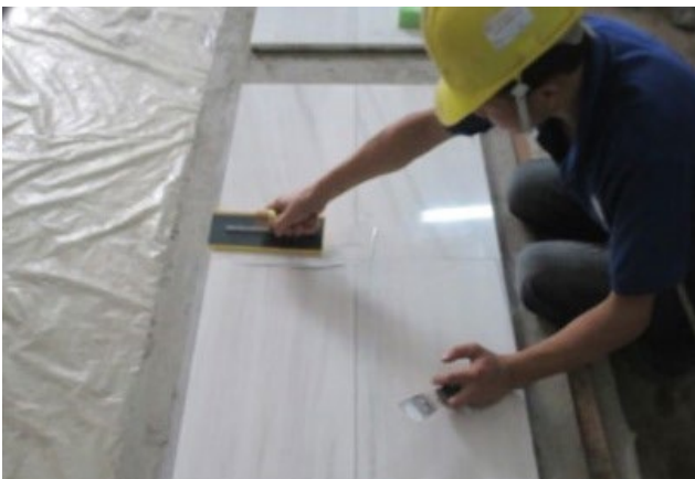
Filling grout joints with firm rubber trowel
