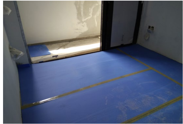
Completed stonework protected with protective material
