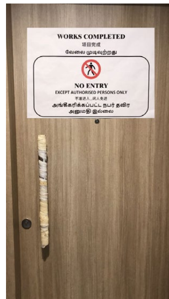
Completed works protected by restricting access
