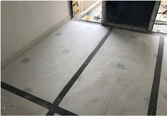
Completed stonework protected with protective material
