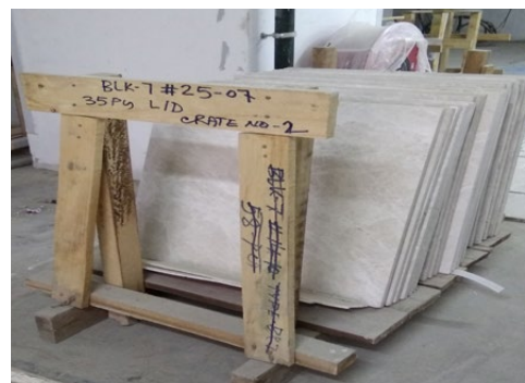
Stones stacked after dry lay
