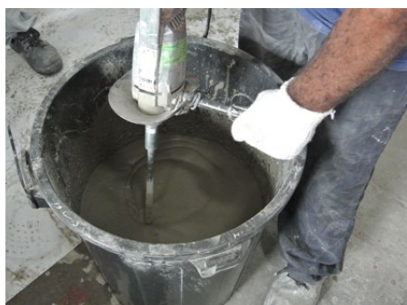
Mixing with an electric mixer
