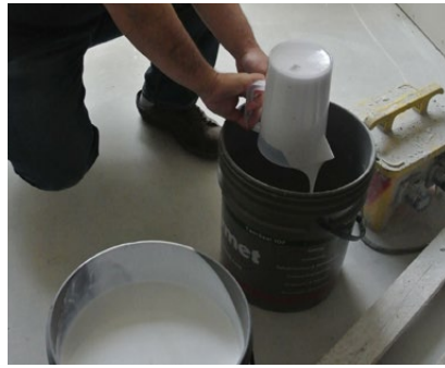
Pouring component 1 into a clean container
