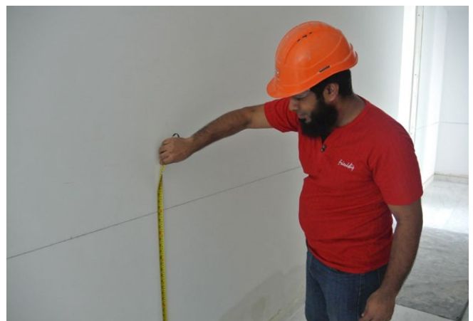
Checking level of surface
