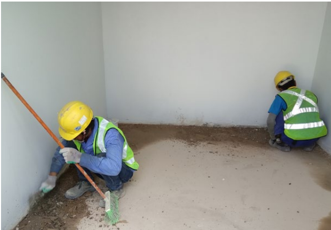
Removing concrete protrusion
