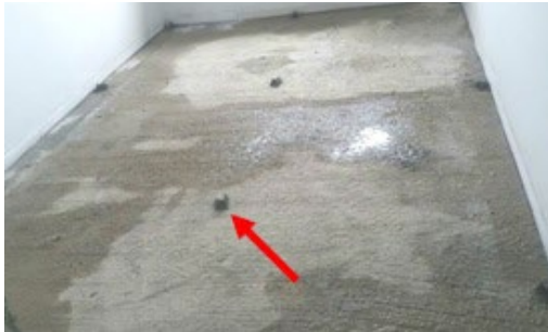
Provide level-pegs before screeding
