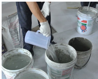
Pouring measured water into clean container
