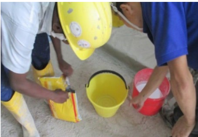
Grout preparation similar to adhesive preparation
