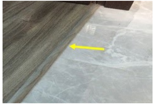
Joint with laminate or timber capping
