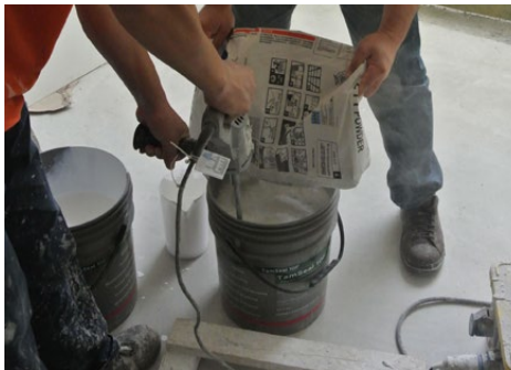
Mixing with electric mixer at low speed
