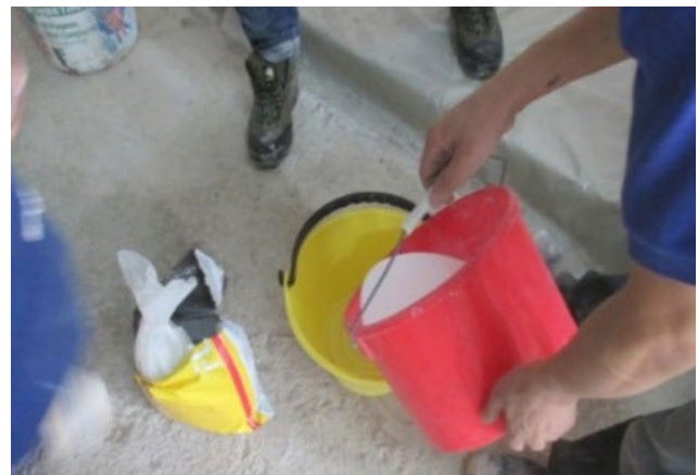
Grout preparation similar to adhesive preparation
