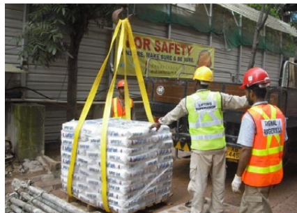
Offloading materials from truck
