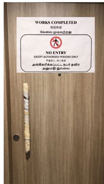
Completed works protected by restricting access
