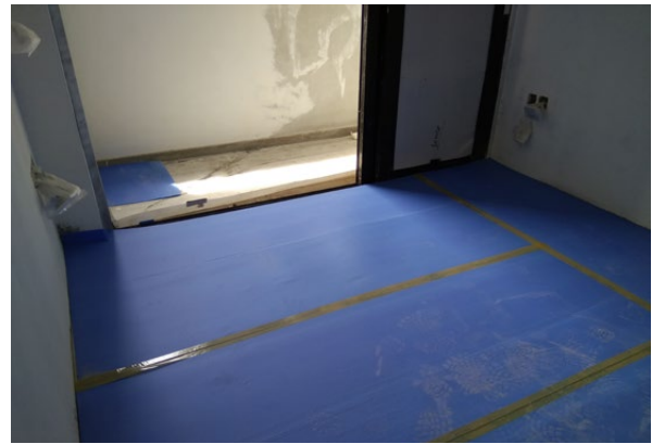
Completed stonework protected with protective material
