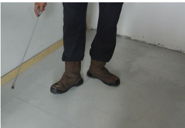
Checking of hollowness
