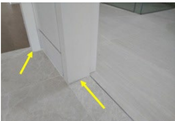
Joint at door frame covered with sealant
