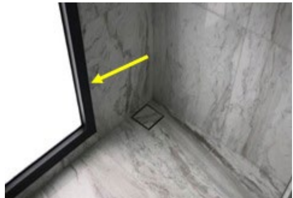
Window frame flush with wall finish surface
