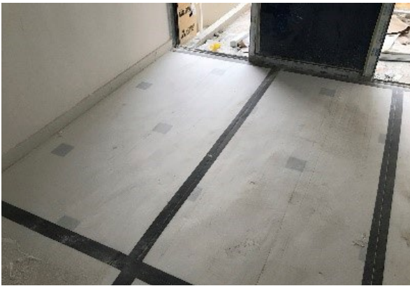
Completed stonework protected with protective material
