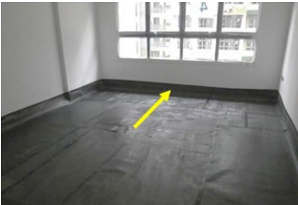
Protection with an up-turn
