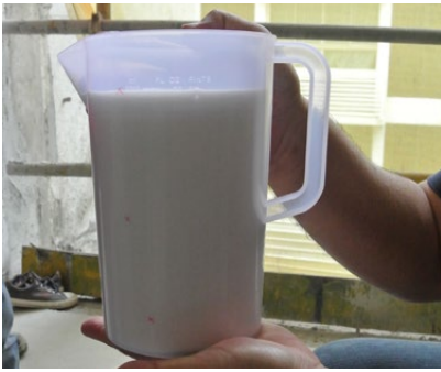
Additive (component 1) in accordance to manufacturer's specs
