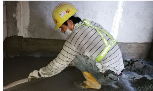
Screeding with timber float
