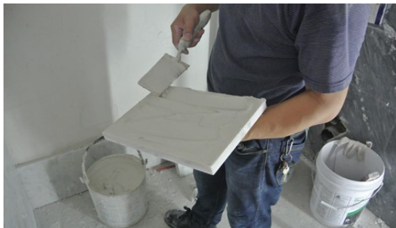
Applying adhesive on back surface of stone
