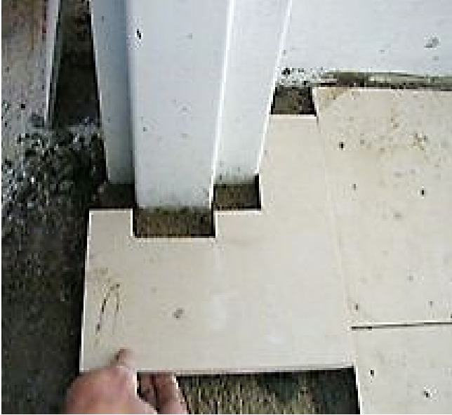
Neatly cut tile at door frame Figure 2.3.1.a
