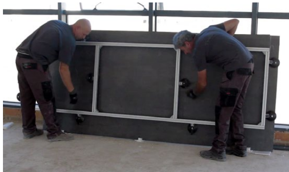
Handling of large format tile using frame
