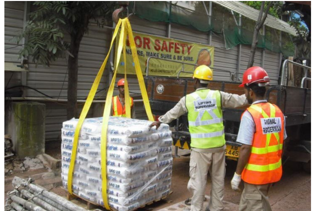
Offloading materials from lorry crane Figure 3.1.b
