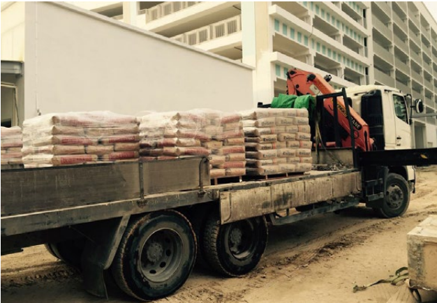
Transporting materials to site Figure 3.1.a
