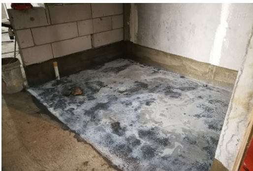
Apply a layer of slurry bond coat using brush or roller and lay screed mortar immediately Figure 4.2.1.c
