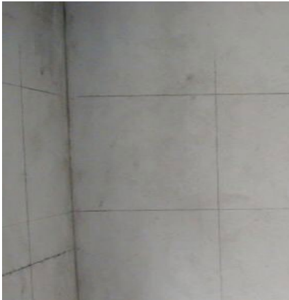
Wall tile setting out Figure 4.3.a
