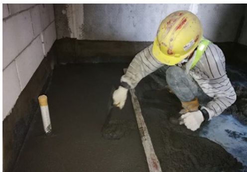
Finishing up the screeding works Figure 4.2.1.e
