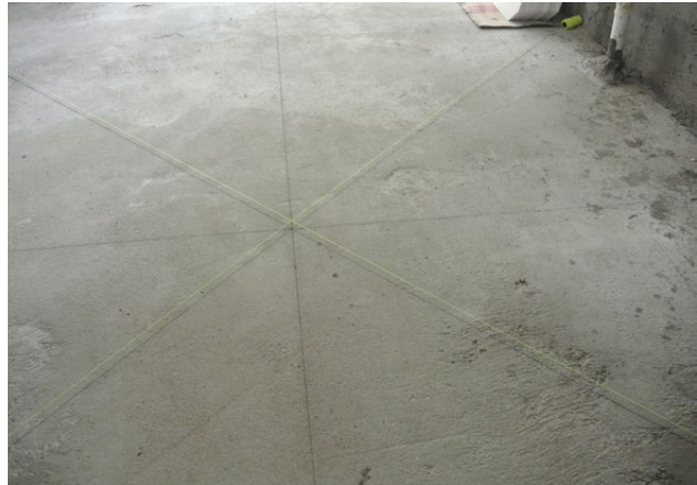
Floor tile setting out Figure 4.3.b
