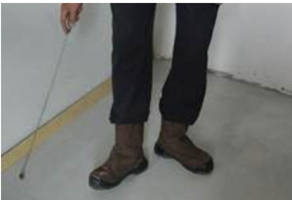
Checking substrate hollowness Figure 4.1.e
