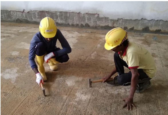
Removing concrete protrusion Figure 4.1.a
