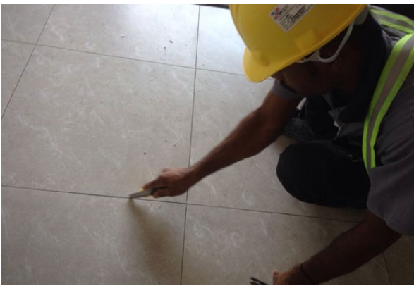
Surface preparation to receive grout mix Figure 5.3.a
