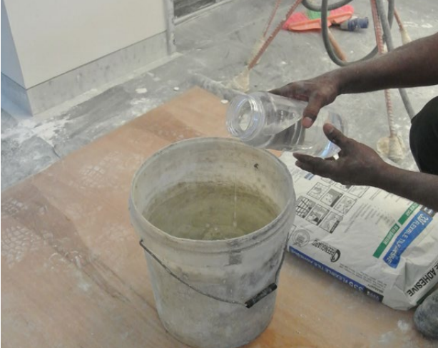
Amount of water or liquid latex added according to manufacturer's specs Figure 5.1.a
