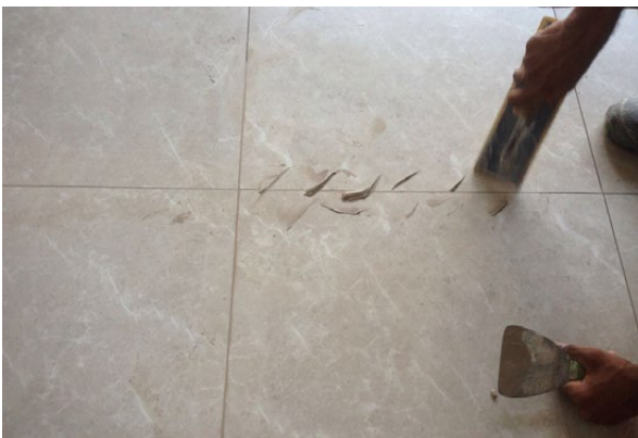
Filling of grout joints Figure 5.3.c
