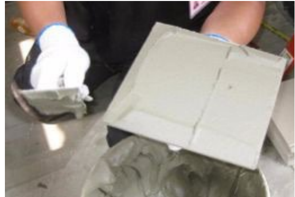
Applying adhesive on back surface of tile Figure 5.2.j
