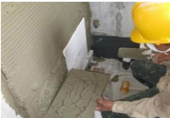
Installing tile on wall Figure 5.2.k
