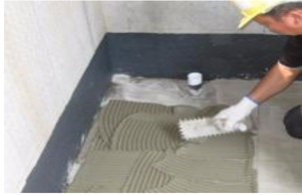
Trowelling adhesive with notched trowel Figure 5.2.b
