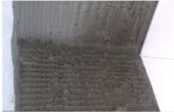
Checking adhesive coverage during tiling Figure 5.2.f
