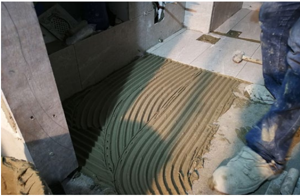
Adhesive fully trowelled Figure 5.2.c
