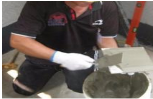
Applying adhesive on back surface of tile Figure 5.2.d
