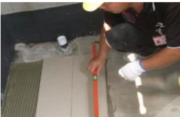
Checking the evenness and lippage after laying each tile Figure 5.2.g
