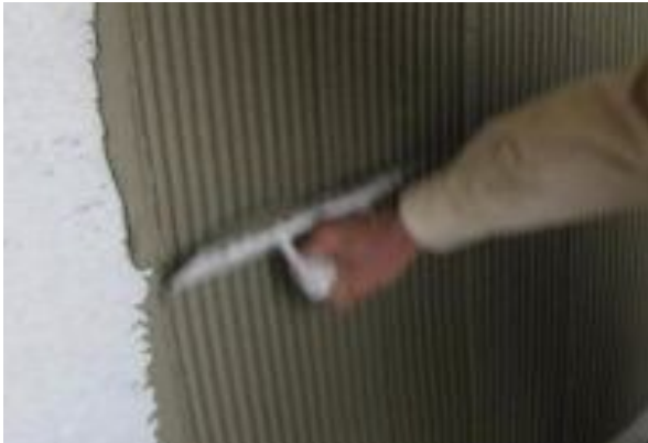
Applying adhesive with notched trowel on wall Figure 5.2.i
