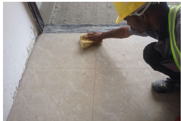
Removal of surplus grout Figure 5.3.d
