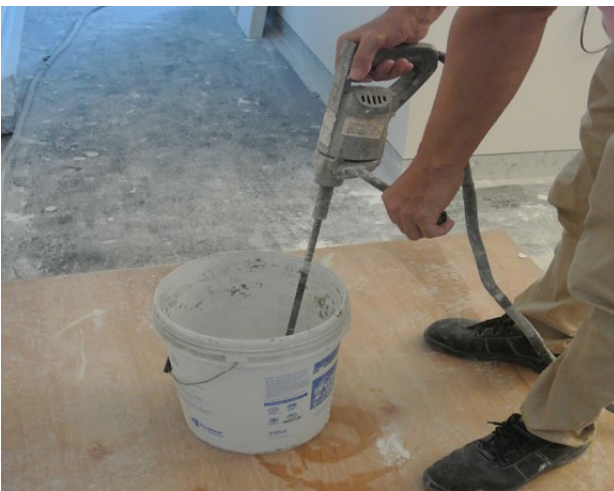
Mix with electric mixer Figure 5.1.c
