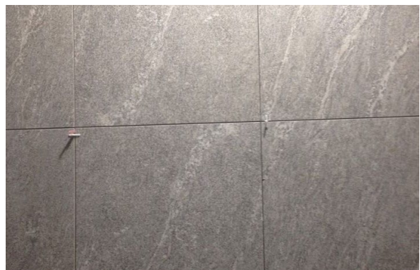
Plastic spacer for consistent joint Figure 5.2.h
