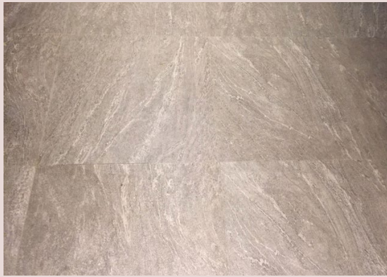
Good surface finishes Figure 5.5.e
