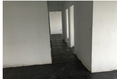
Laying of protection over completed floor tiles Figure 6.b
