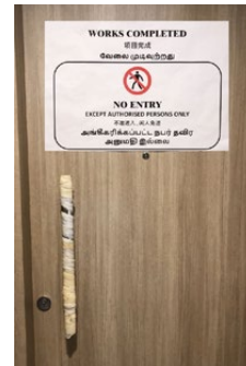
No entry to prevent damages to completed tiles Figure 6.d
