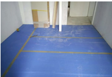
Laying of protection over completed floor tiles Figure 6.c
