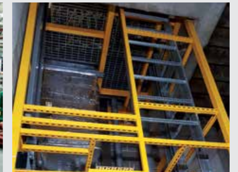
Prefabricated Riser Module Photo credits: Laing O'Rourke
