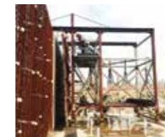
Moveable Lifting Frame Wall Formwork
