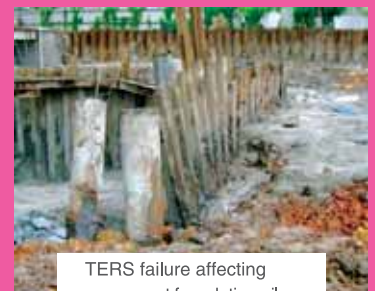
Anchorage failure
