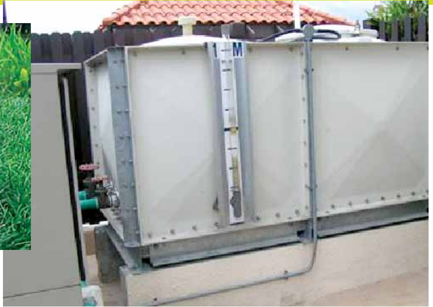
Rainwater tanks can be sealed tanks designed to contain rainwater collected from roofs.
