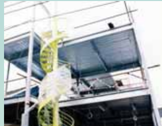
Structural steel frame with bondek decking was used for the house.
