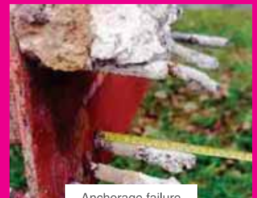
Anchorage failure
