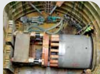
Seletar Link Sewer Contract 1
