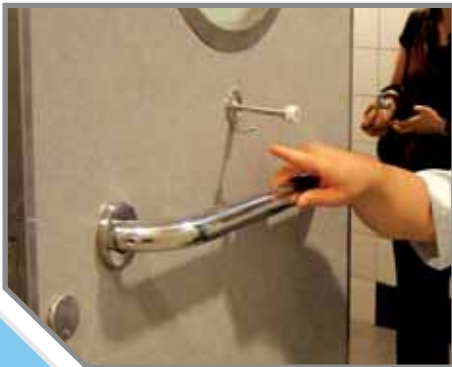
Clothes hook in accessible toilet at useable height
