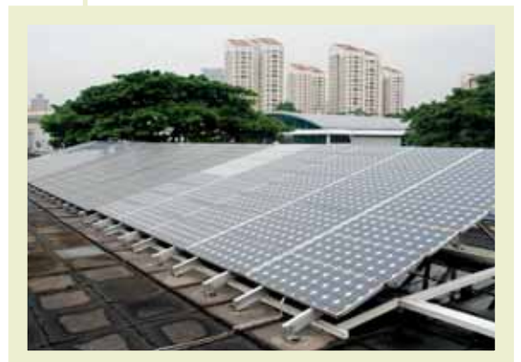
Three types of photovoltaic systems - mono-crystalline, poly-crystalline and thin film (CIS) - are installed at the BCA Academy.
