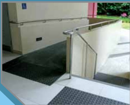
Warning tactile indicators at top and bottom of stairs
